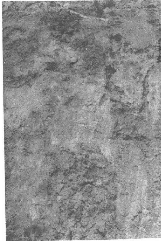
Figure A7. Detail of a portion of the east wall of the excavation. See Figure A2 for location.
