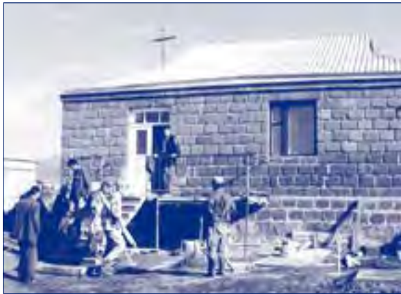
In Yerevan, Armenia, an Armenian family prepares to move into a house constructed with the help of a USAID-sponsored housing program.
