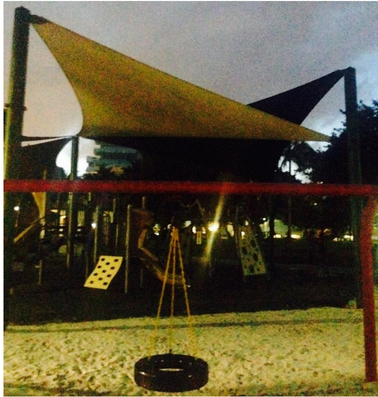
Figure 13 Triangular Flap of Shade Attached to Pole in Center and on Sides
