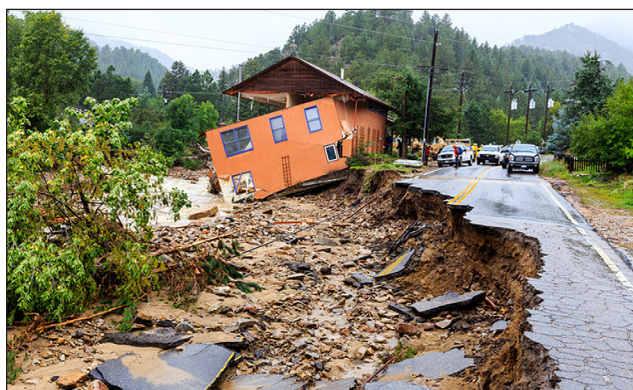
Flooding from heavy rains damaged Boulder, Colorado, in September 2013—one of several extreme events examined in the collaborative report. (Source: S. Zumwalt, FEMA)
