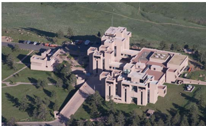
Aerial view of the National Center for Atmospheric Research (NCAR) Mesa Laboratory. NCAR provides the university research and teaching community with tools such as aircraft and radar to observe the atmosphere and with the technology and assistance to interpret and use these observations, including supercomputer access, computer models, and user support. Credit: © University Corporation for Atmospheric Research
