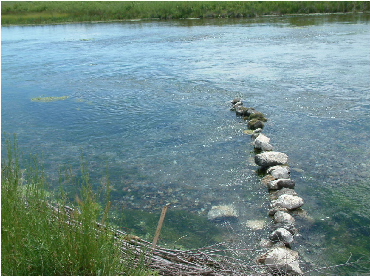
Figure 12. Rock deflector immediately below sloping sites.
