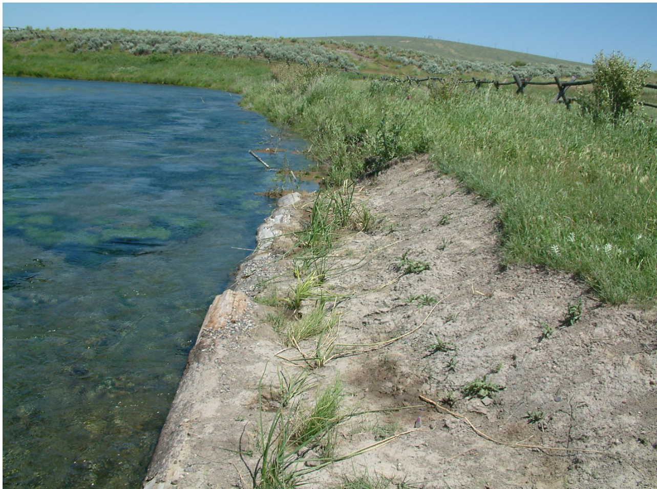
Figure 4. Sedge and bulrush planted on sloping at Head-end Spring Creek.
