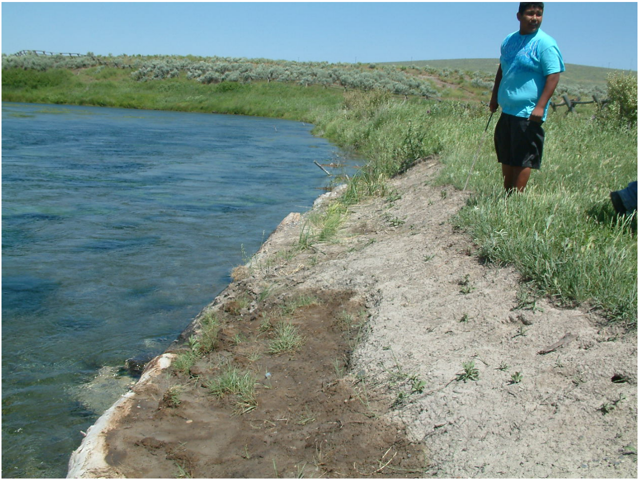
Figure 11. Sloped and planted streambank at Head-end site 2009.
