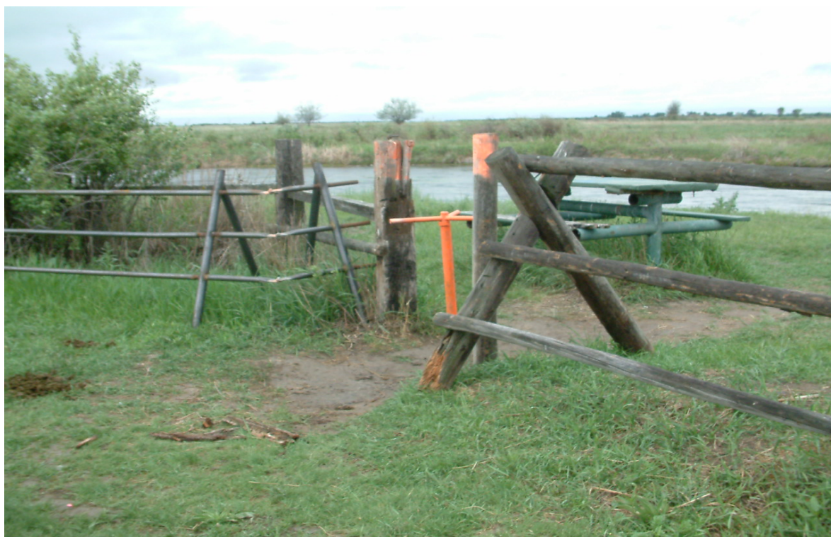
Figure 5. Steel jack and rail and access point at Head-end Spring Creek 2009.
