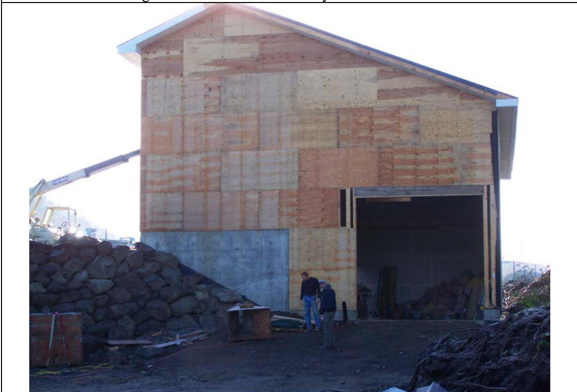
Framing of North wall. Note mechanical room door. October 2007
