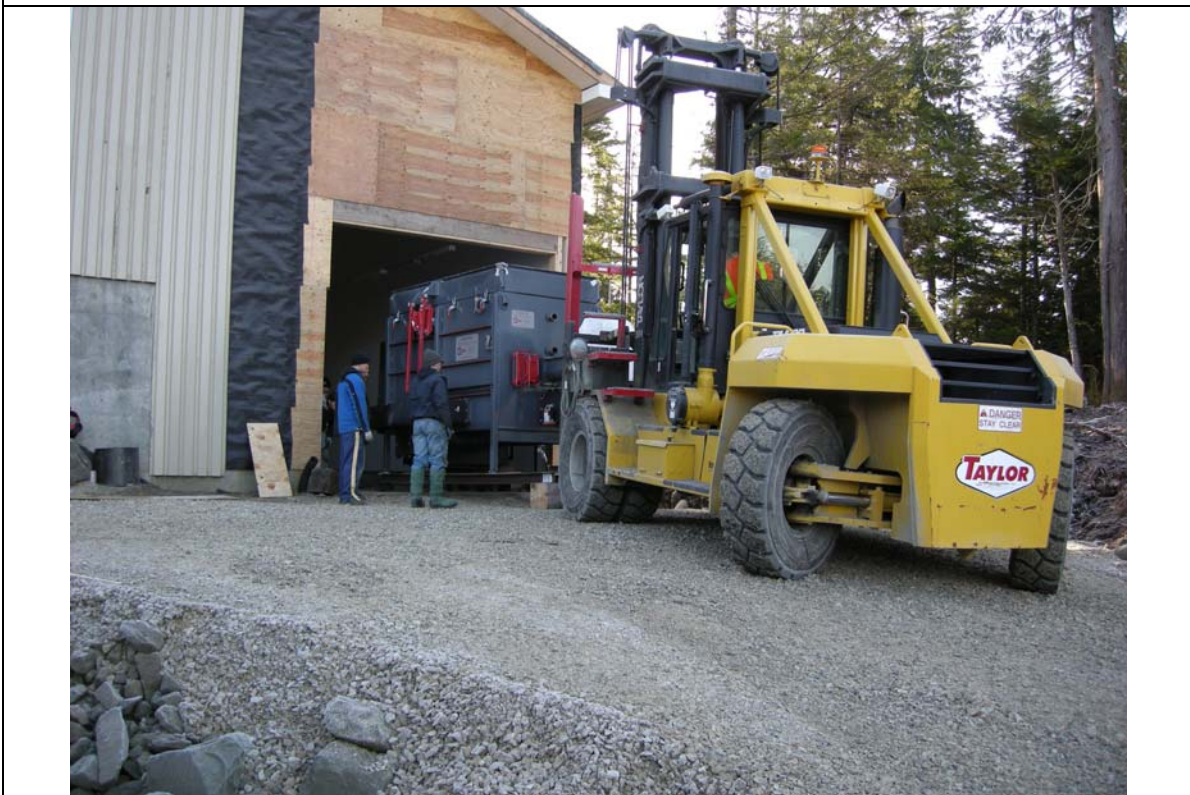
Placement of gasifier into mechanical room. November 2007.
