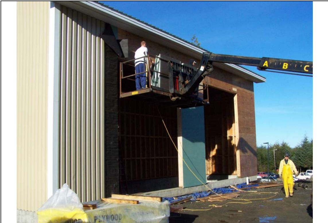
Siding of east wall at fuel delivery doors. October 2007
