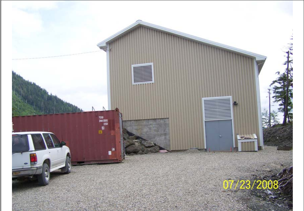
Substantially complete north wall of boiler building.
