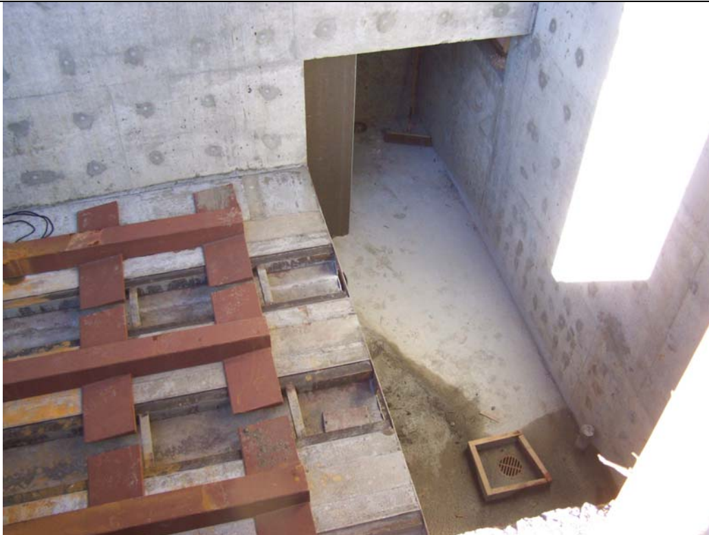
Auger pit at north end of wood bin. October 2007.
