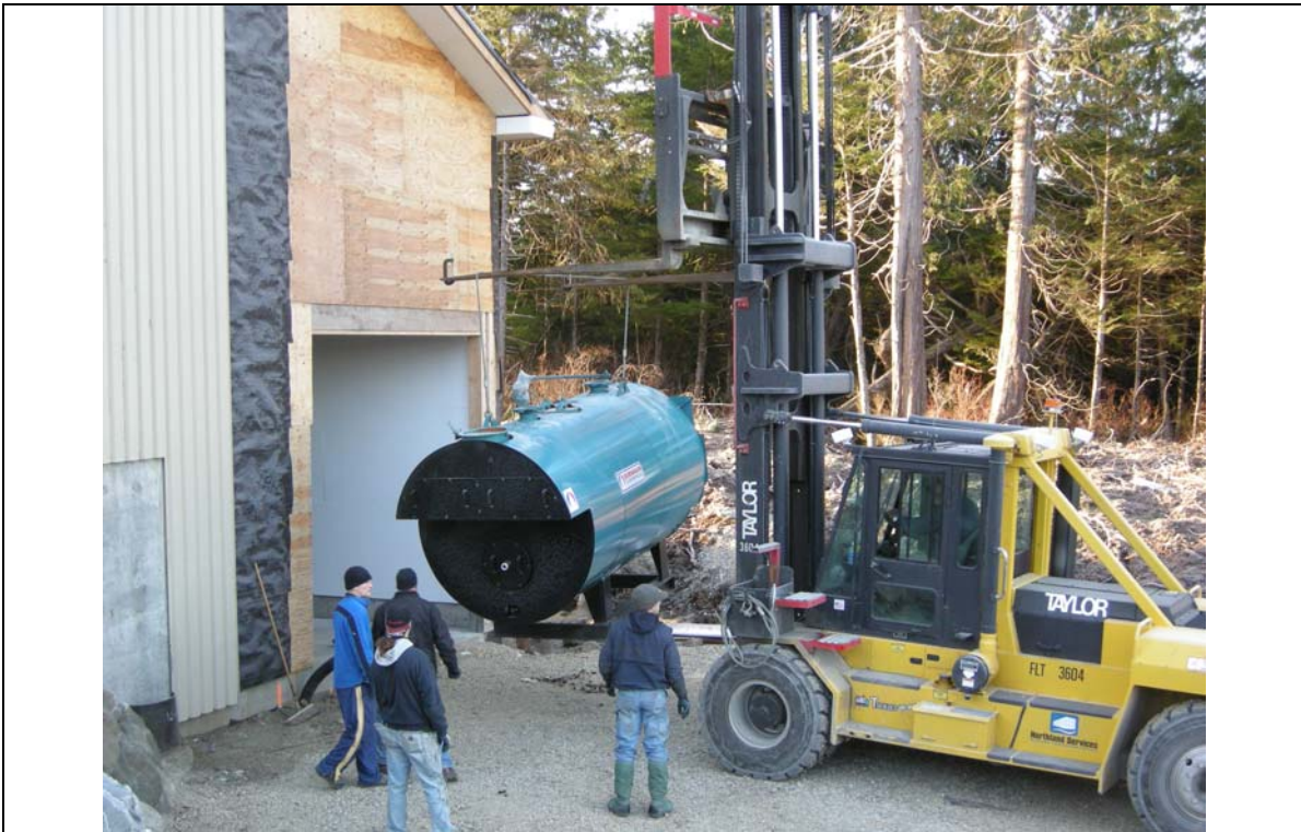
Placement of boiler into mechanical room. November 2007
