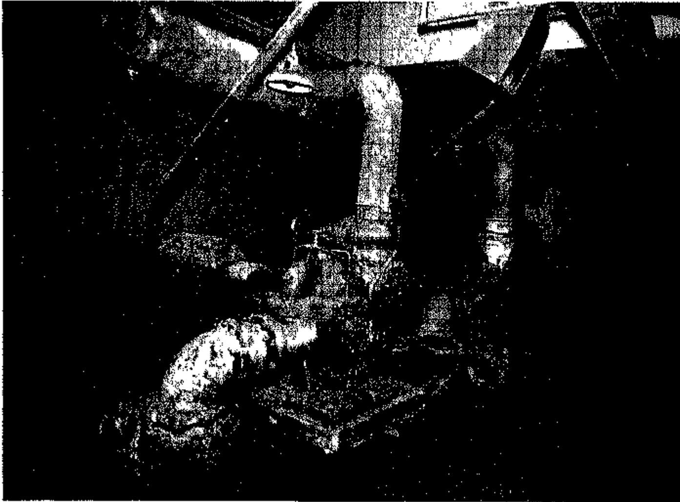
Fig. 38. K-706 Water Pump House Service Water Pumps are Insulated with 1-1/2" - 2" of Asbestos
