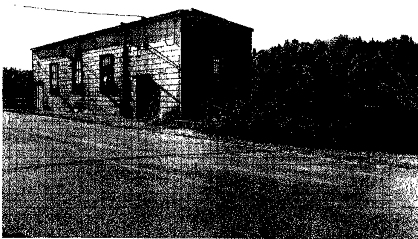
Fig. 8. K-705 Water Intake Building East Side of Building
