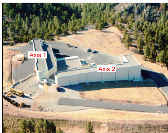
Figure 1 Areal View of the DARHT Facility
