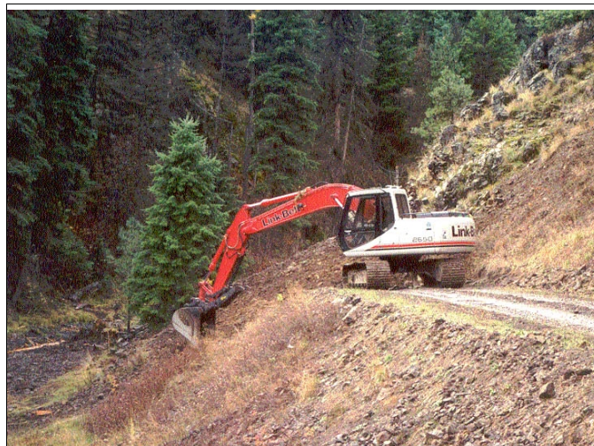
During project: Recontouring drawbottom road. Photo from USFS.
