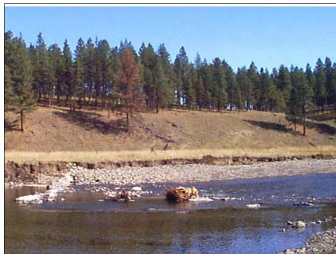
Post-project: Vortex rock weir with 2 root wads.
