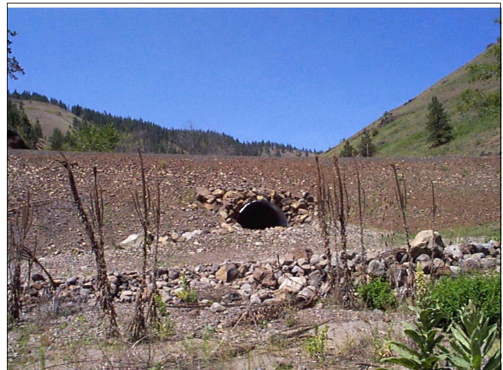
Post-project: Showing bottomless arch culvert.
