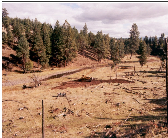
Meadow Creek during project: showing railroad grade removal and lack of riparian vegetation. Photo from ODFW.
