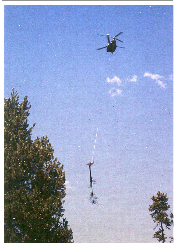
Helicopter transporting whole tree for placement in stream.
