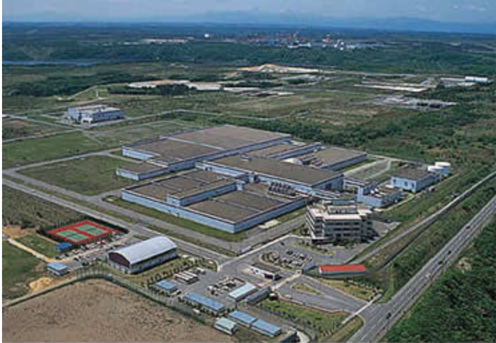
Fig. 22. Rokkasho Uranium Enrichment Plant, Japan. Source: japannuclear.com
