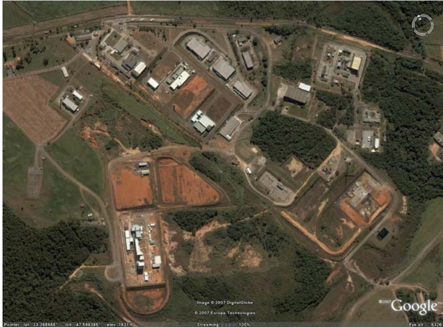
Fig. 24. Aramar Experimental Center, Brazil. Source: Google Earth
