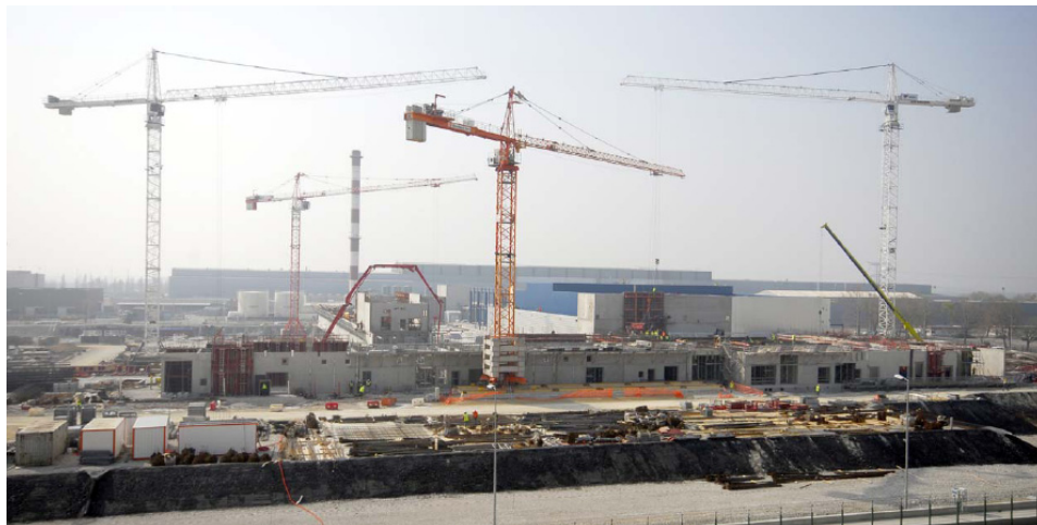
Fig. 17. Georges Besse II plant under construction, March 2007. 54
