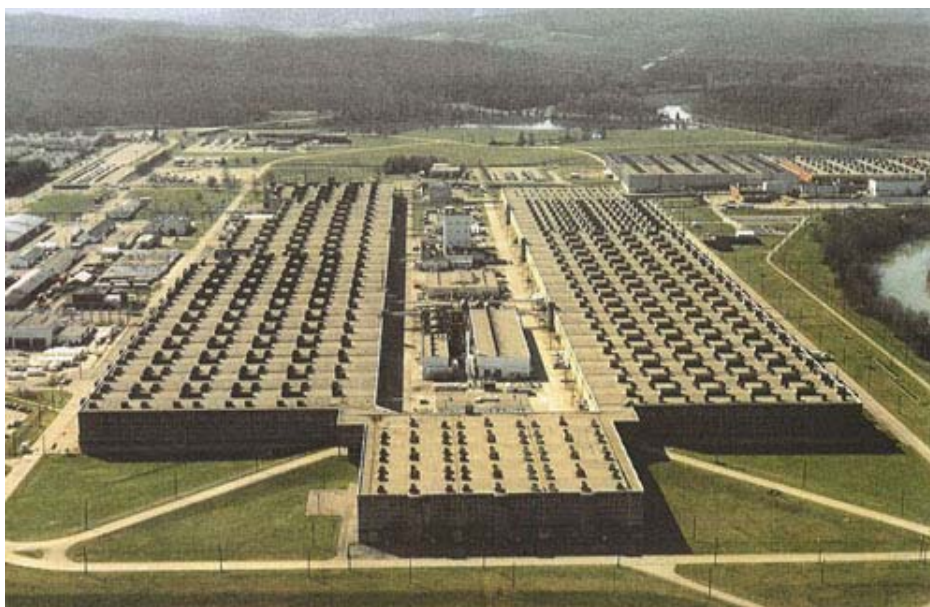
Fig. 2. K-25 building at the now-dismantled Oak Ridge GDP, United States.
