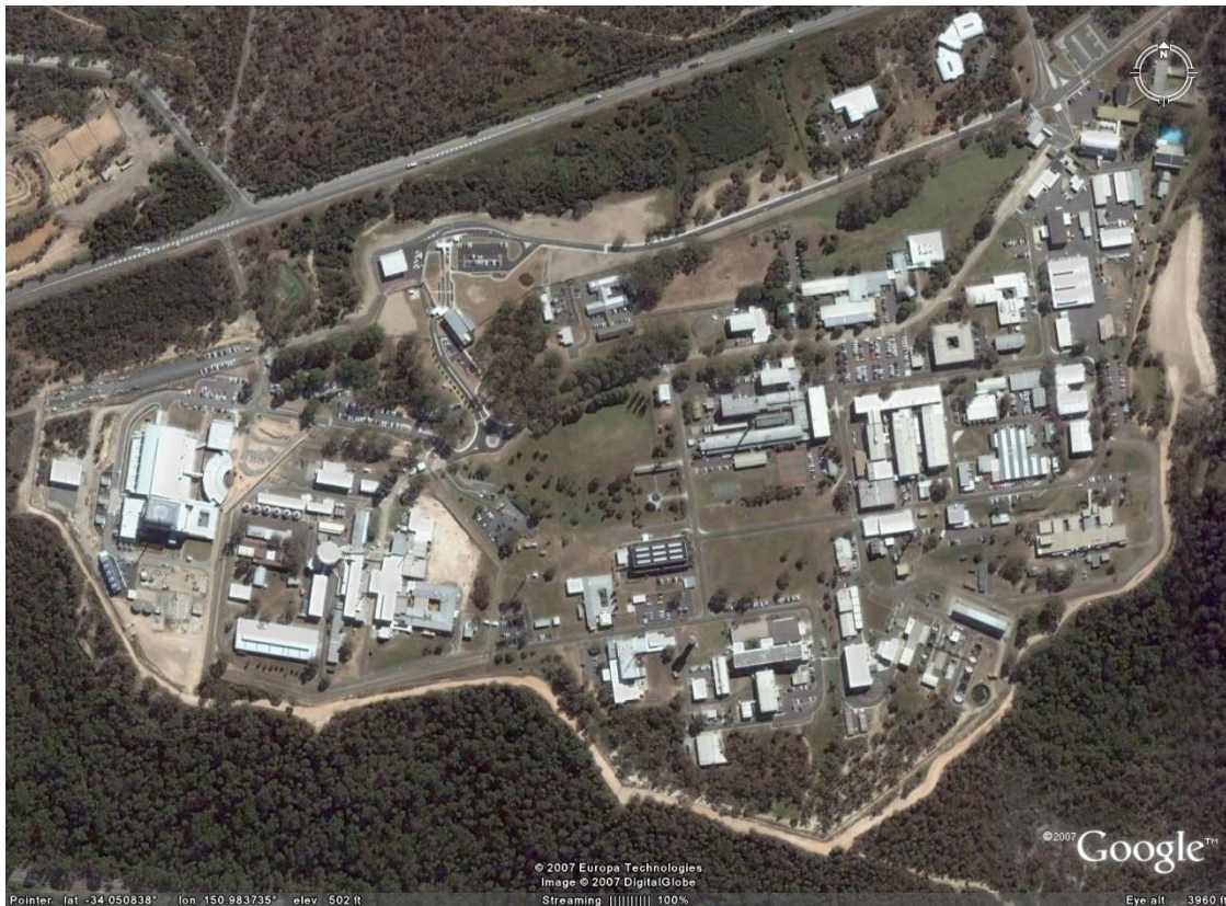
Fig. 23. Lucas Heights Science and Technology Centre, Australia. Source: Google Earth
