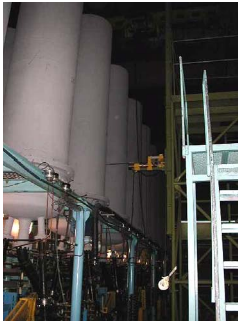
Fig. 27. Argentine diffusers, Pilcaniyeu. Source: Whitaker, 2005 109
