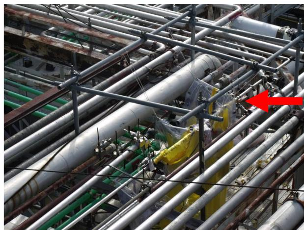
FIGURE 2 – Installed A-Line Hot Taps
