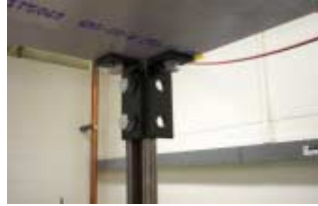
Figure 2. Photo of a joint on the structure.
