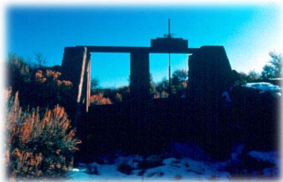
Figure 16. Headgate from early 1900s irrigation project in the area now known as INL.
