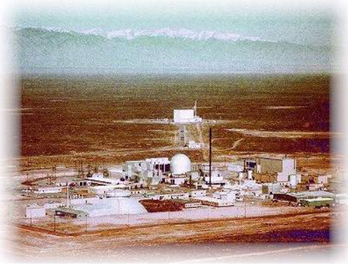
Figure 24. Aerial view of MFC.
