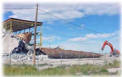
Figure 22. Demolition of the WRRTF stack.
