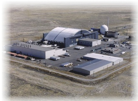
Figure 21. Aerial photo of the LOFT facility (demolished in 2006) and ANP hangar at TAN.
