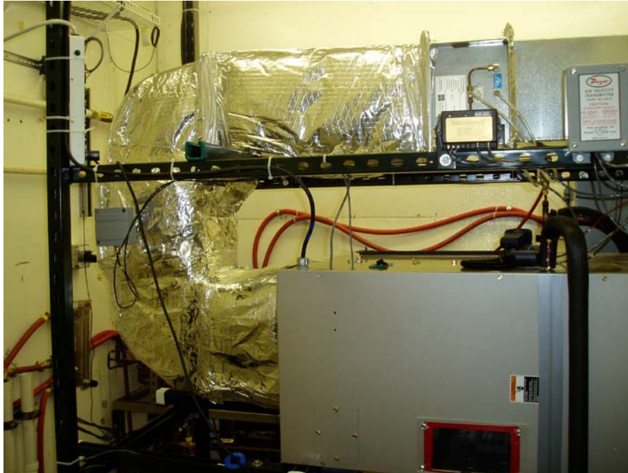
Fig. 3.11. Air supply duct and flow station arrangement.
