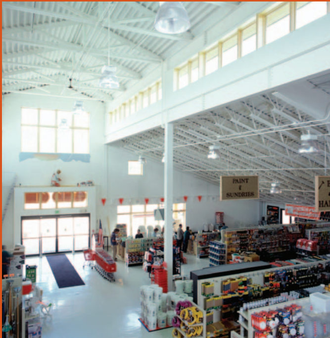
The BigHorn Home Improvement Center, a retail complex in Silverthorne, Colorado, is an example of a retailer using natural daylighting to reduce energy use. Credit: Jim Yost/PIX 09218
