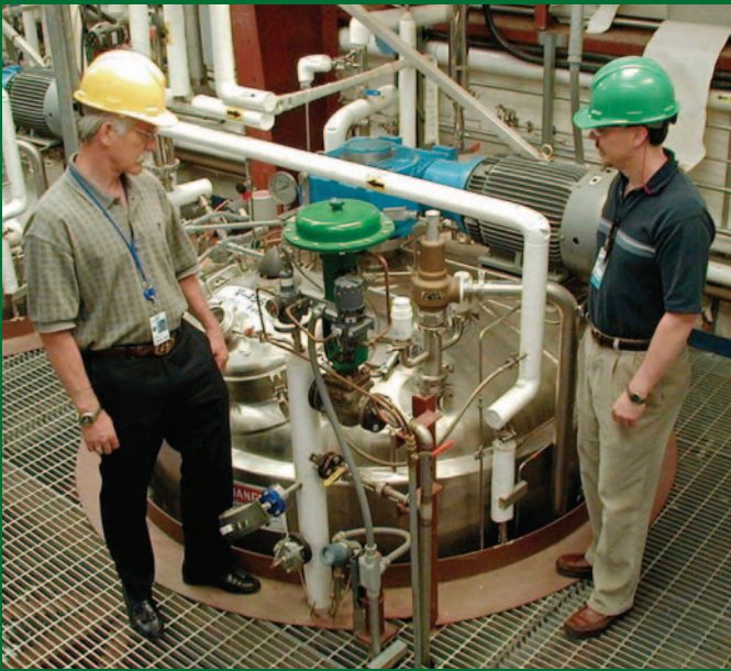
NREL's John Ashworth, left, and Dan Schell inspect a fermentation tank in the lab's Alternative Fuels User Facility pilot plant. DuPont and NREL researchers worked side-by-side in the facility to move biomass conversion technology from the laboratory to pilot scale. Credit: Nick Nagle/PIX 13486
