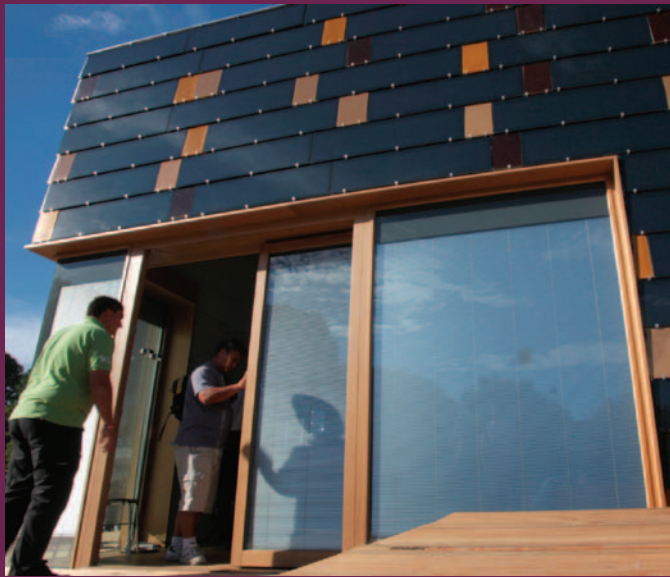
Team Germany's winning "Cube House" featured silicon and thin-film solar panels on all visible sides of the house. The design's solar panel operates a toy on the front porch of the home. Credit: Stefano Paltera/U.S. Department of Energy Solar Decathlon/PIX 16893
