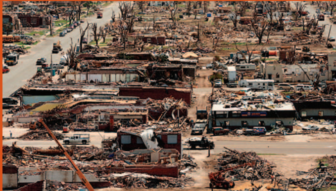
A tornado on May 4, 2007 destroyed 90% of Greensburg, Kansas. With NREL's help, the city is rebuilding to stringent energy efficiency standards and adding renewable energy sources in an effort to be the nation's greenest community. PIX 16290
