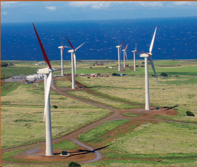
A 10.5 MW wind farm near the northern tip of Hawaii's Big Island has been generating electricity since 2006. Courtesy of Hawaiian Electric Light Company (HELCO)/PIX 14697
