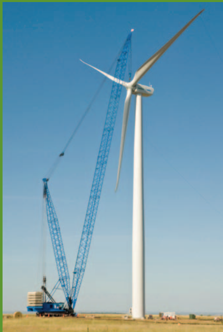
Blue skies and calm conditions contributed to a smooth installation of a General Electric 1.5 MW wind turbine at the National Wind Technology Center. Credit: Pat Corkery/PIX 16570
