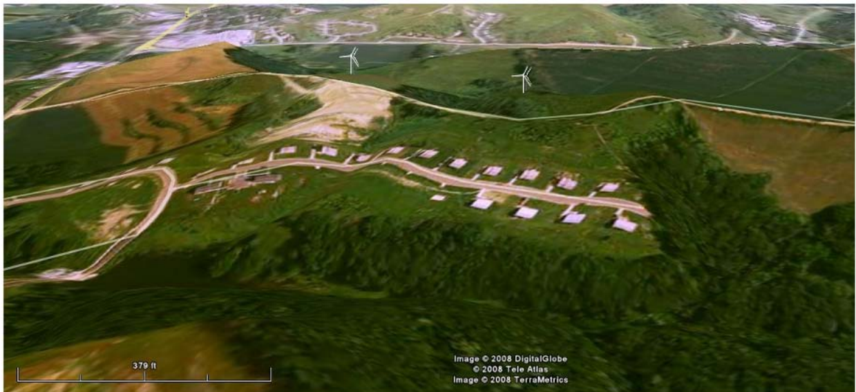
Figure 5.3-2, Kelly Subdivision, Northern View, Post-Construction
