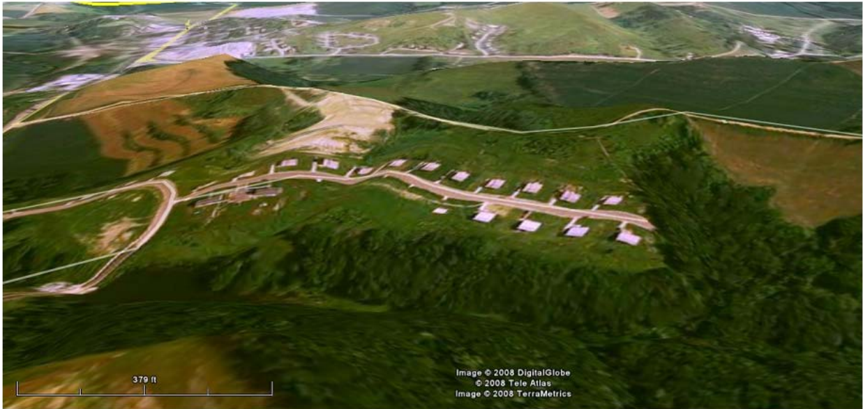
Figure 5.3-1, Kelly Subdivision, Northern View, Pre-Construction
