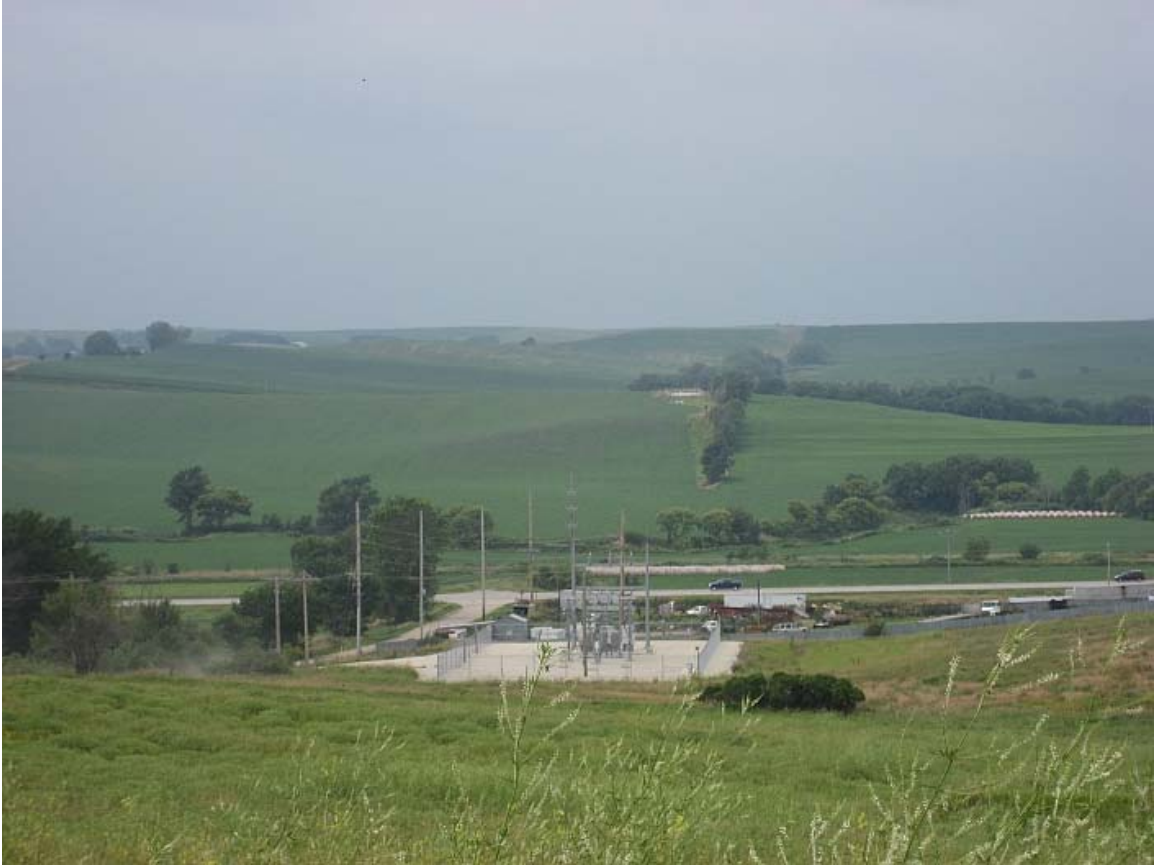
Figure 4.3-4, Looking West Toward Substation
