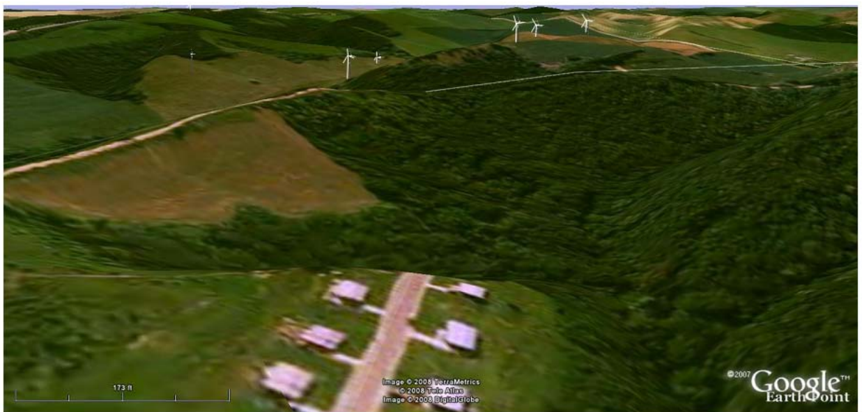
Figure 5.3-5, Kelly Subdivision, South East View, Post-Construction
