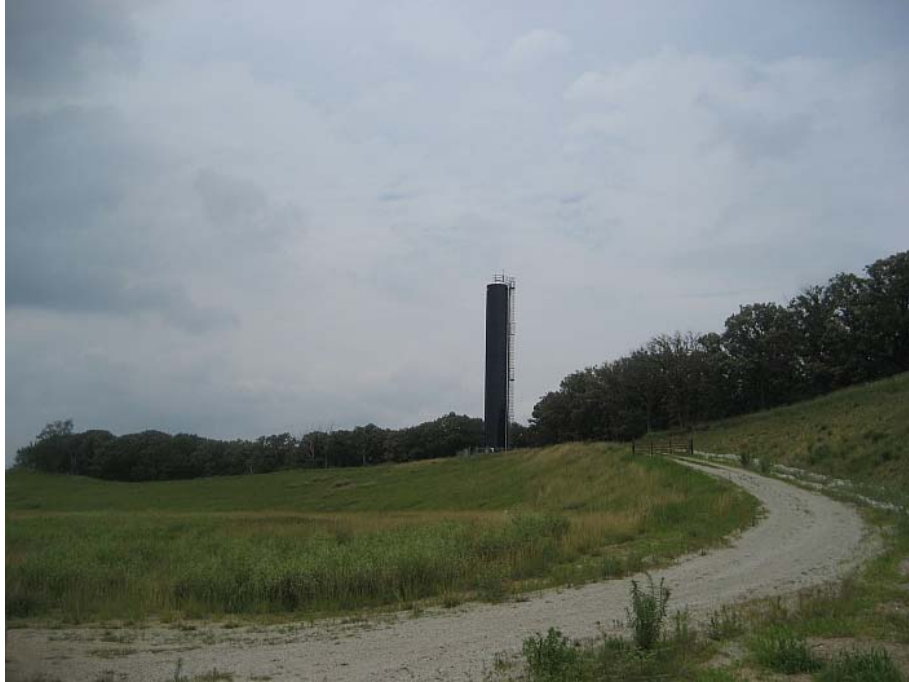
Figure 4.3-6, Looking North Toward Water Storage
