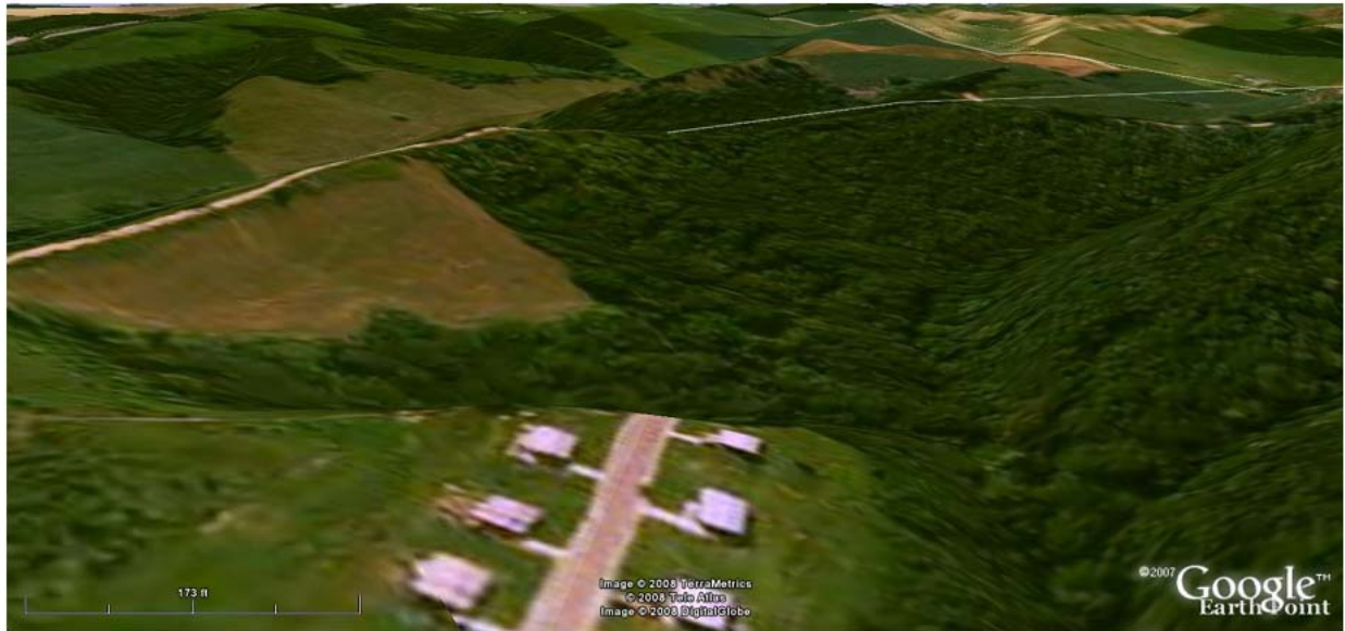
Figure 5.3-4, Kelly Subdivision, South East View, Pre-Construction
