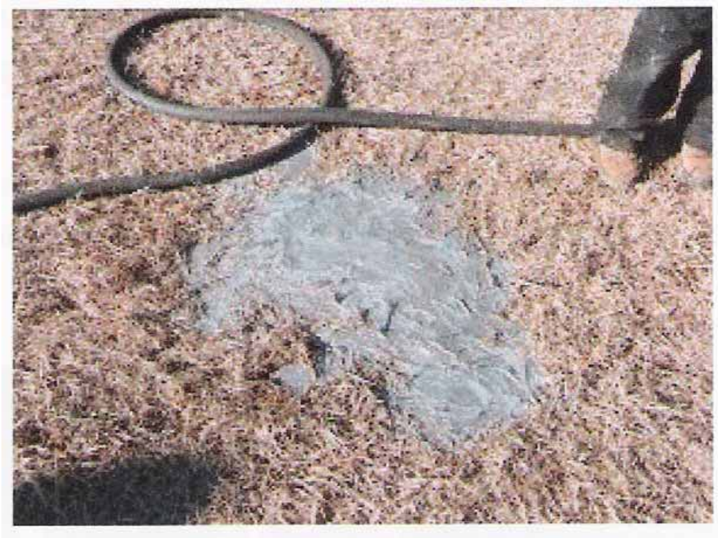
Daylighting of EHC slurry observed in open ground near injection point PT2.
