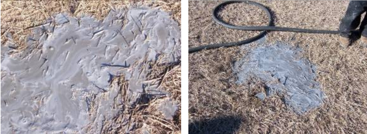
Figure 15: Daylighting at multiple points around PT-14 and PT-2
