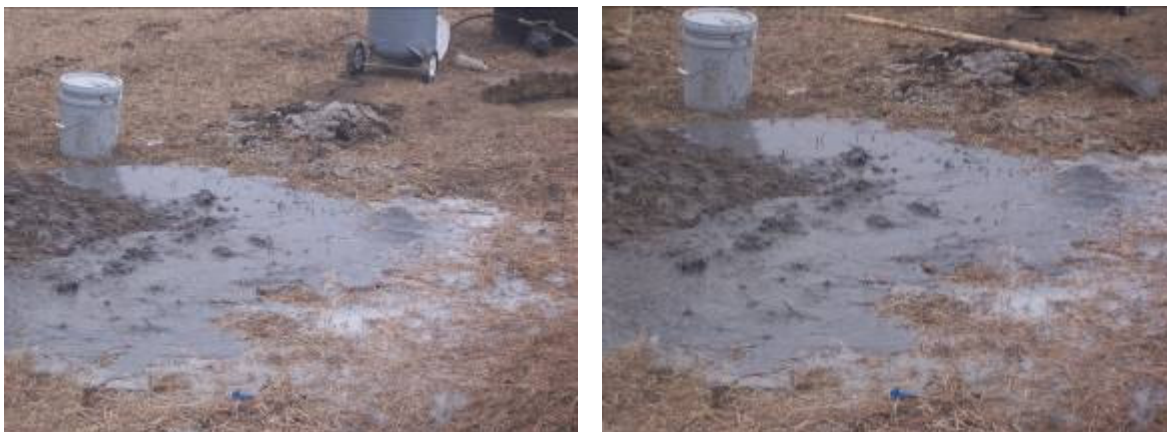
Figure 14: Surficial Daylighting near PT-7 and PT-10
