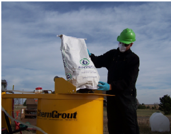
Figure 4. Mixing of EHC and EHC-A on Site
