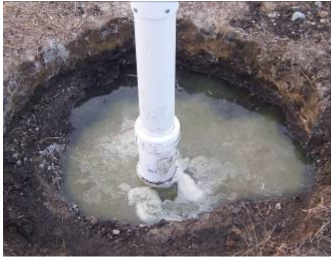
Figure 11. Well Seal Repair at MW-02
