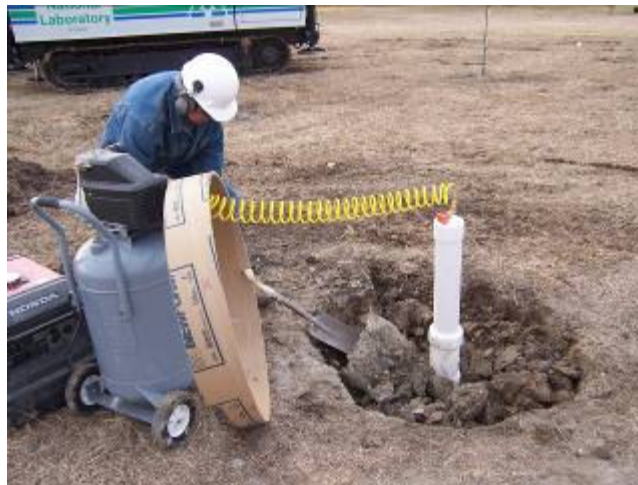
Figure 11. Well Seal Repair at MW-02
