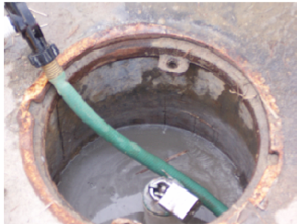
Figure 13: Daylighting at SB07R during injection at PT-6
