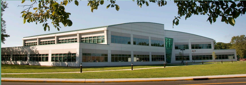
RESEARCH SUPPORT BUILDING
