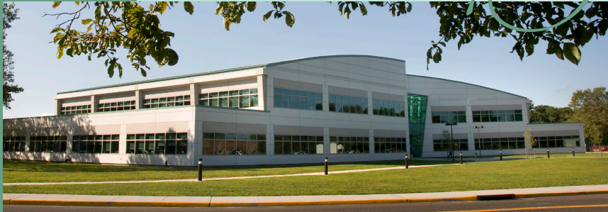
RESEARCH SUPPORT BUILDING
