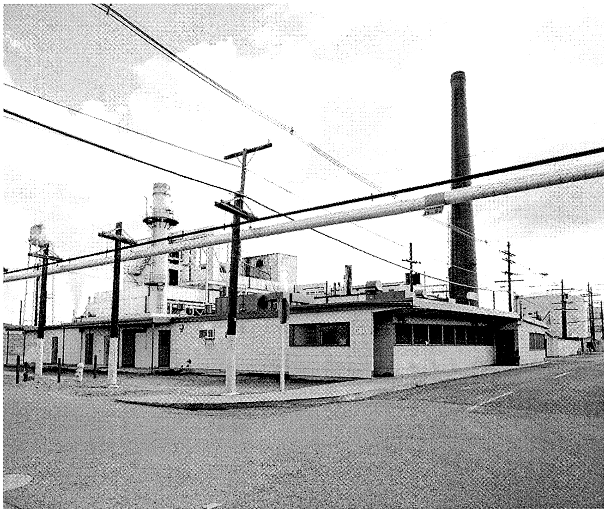
Figure 10. 3707D Information Services Building.
