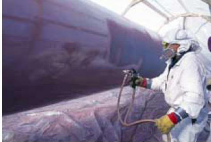
FIGURE 2.1-5 Crew Coating a Pipeline Field Joint (Source: TAPS 2001)
