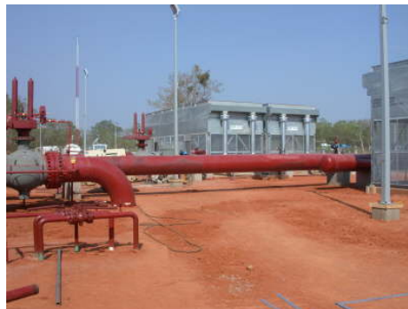
FIGURE 1.2-4 Typical Metering Station (Source: U.S. Pipeline, Inc.)
