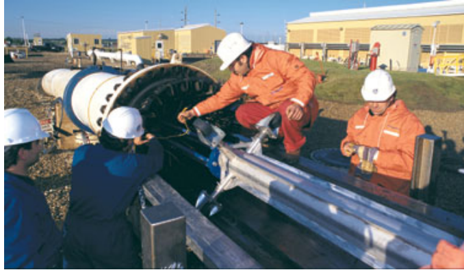
FIGURE 1.2-7 Crew Inserting a Pig into a Pipeline (Source: Argonne Staff)
