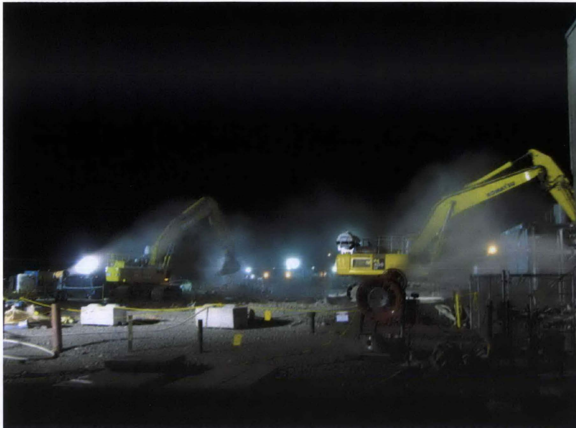
Fig. 2. Nighttime demolition operations
