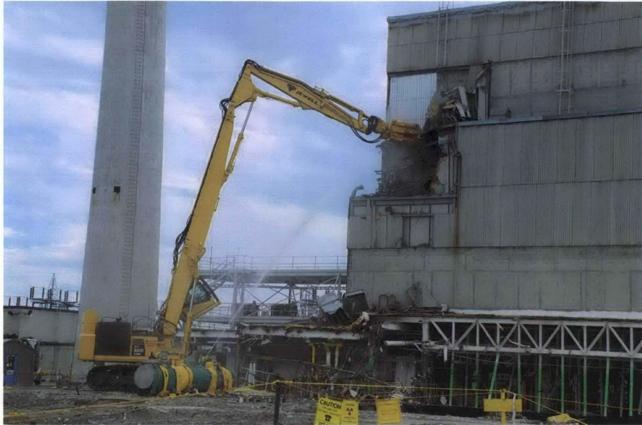
Fig. 3. High-reach excavator demolishing the F-G (reactor interface area) area
