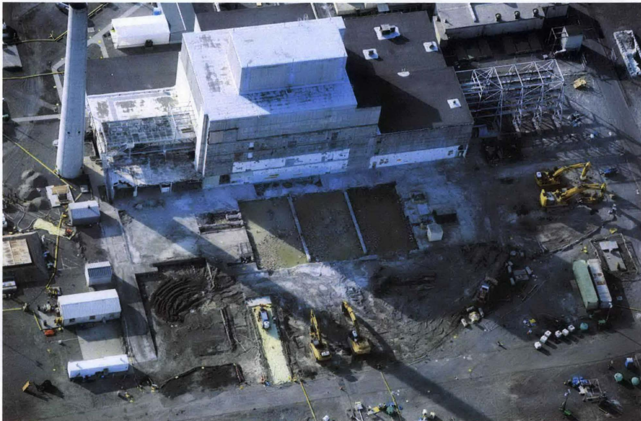
Fig. 4. Superstructure demolition complete.
