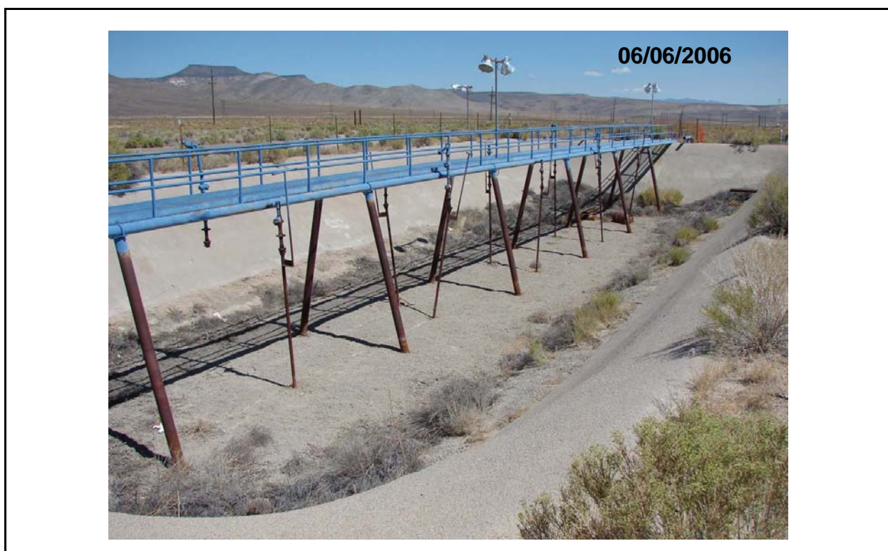
Figure A.3-1 Corrective Action Site 02-09-48
