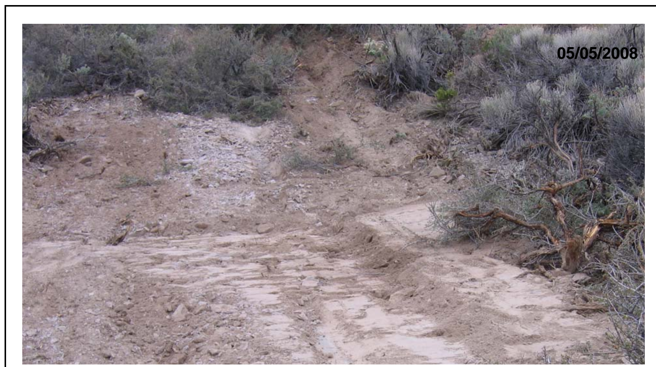
Figure D.1-6 Area after Pipe Debris Removal at CAS 12-09-01
