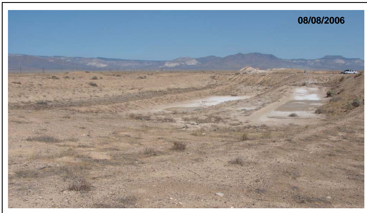
Figure A.4-1 Mud Trenches in Southern Footprint
