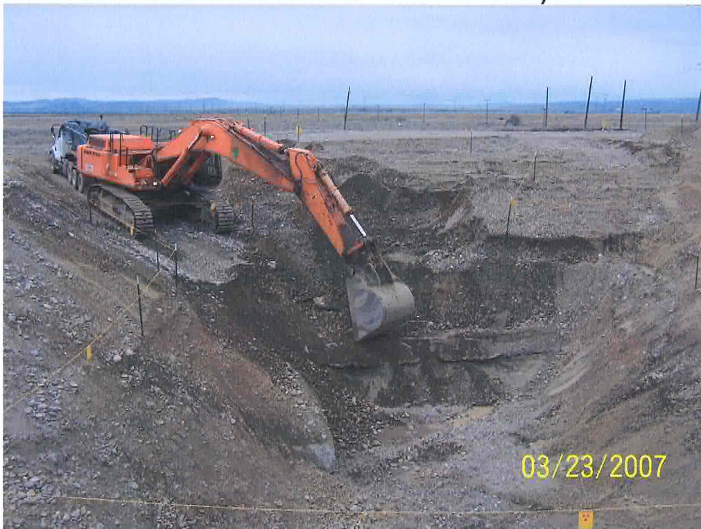
Excavating pipe encased in concrete. (Looking southwest; near bottom of 118-F-8:4 waste site.)
