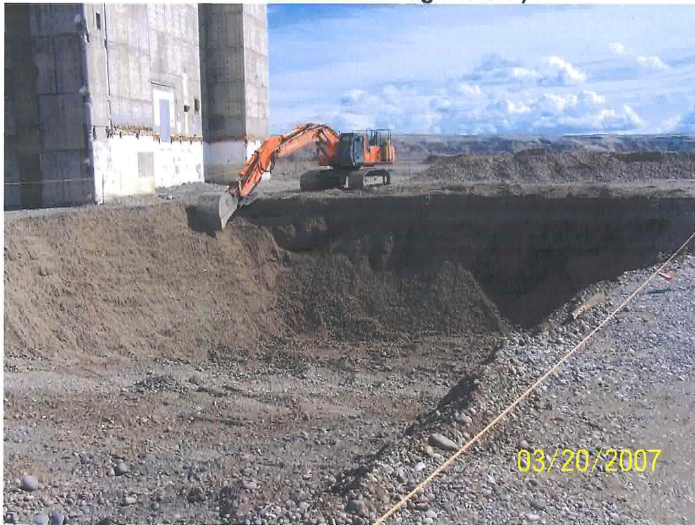
Excavating pipe encased in concrete. (Looking southwest; near bottom of 118-F-8:4 waste site.)
