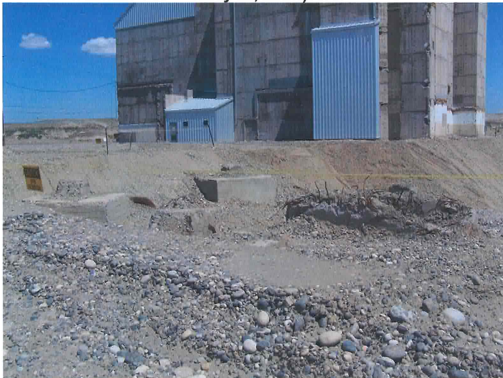
100-F-26:14/118-F-8:4 waste sites. (Looking northeast; May 24, 2007.)
