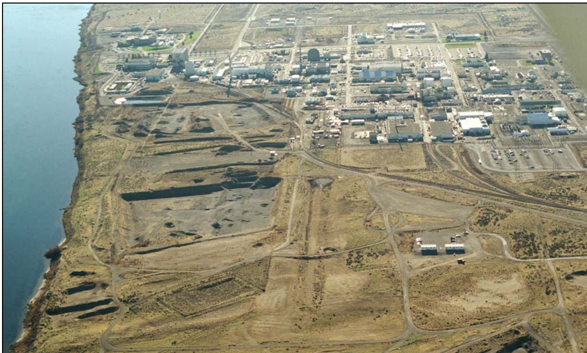
Figure 1.4. Open Excavations at the 300 Area
