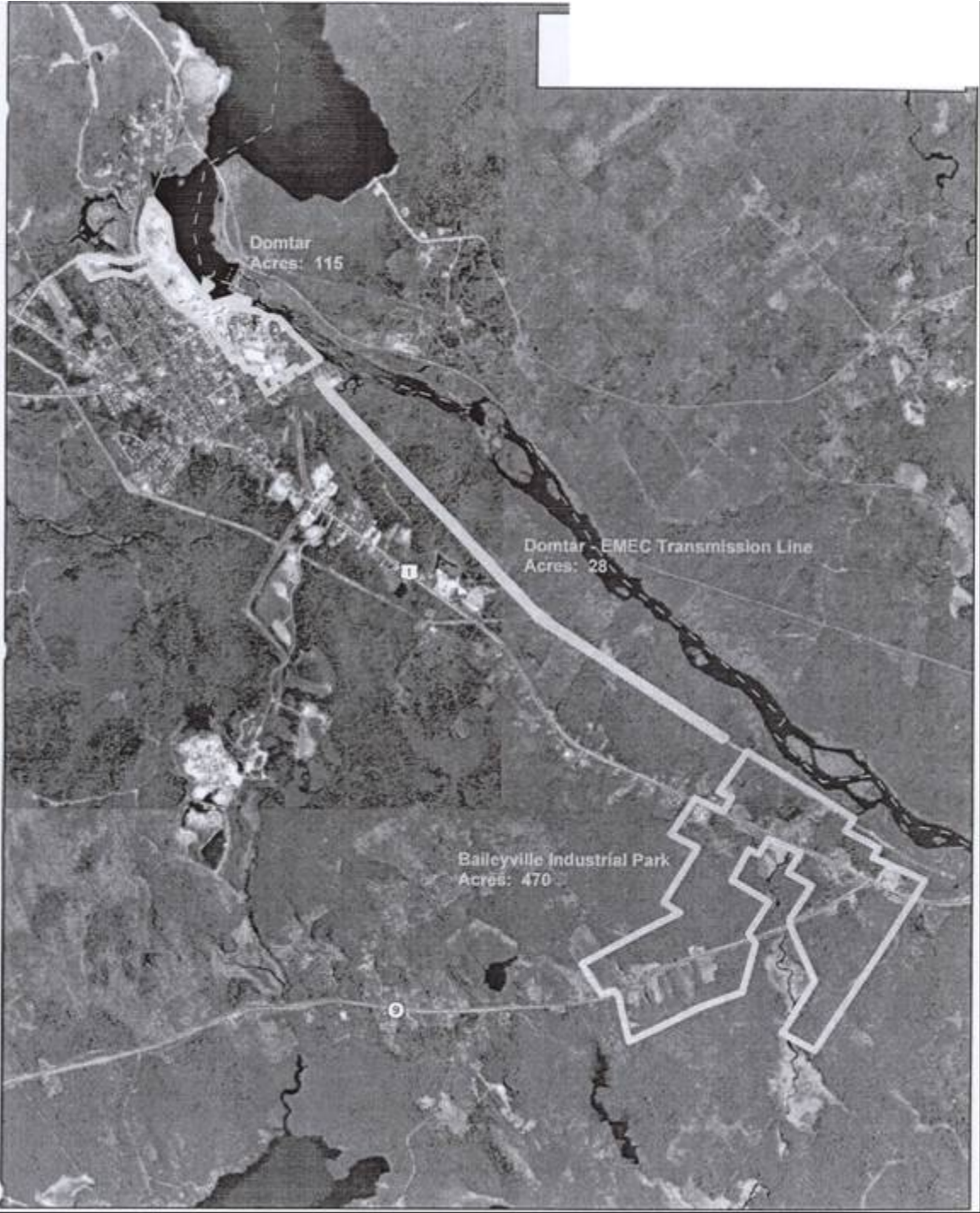
Baileyville, Maine. Domtar and Baileyville Industrial Park
