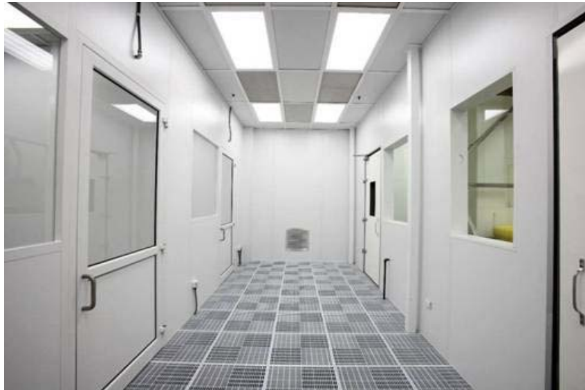
Fig. III-4. The common clean anteroom of the joint ANL/FNAL SCSPF. An additional pair of class-100 clean areas (not shown) lie through the doors to the left of the figure.
