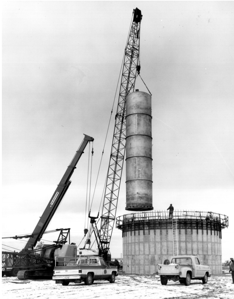
Figure A-5. Installation of Bin VES-WS4-142 in Calcined Solids Storage Facility IV (76-4518).
