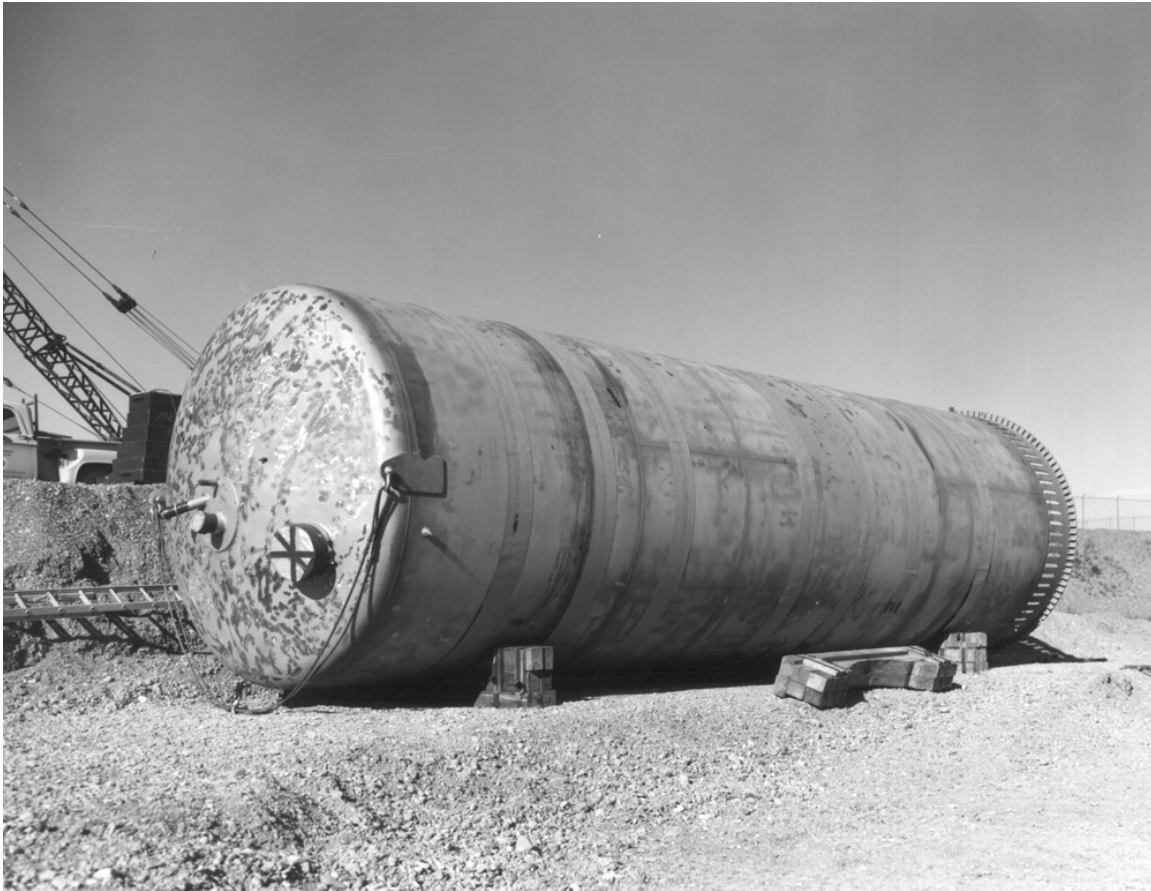
Figure A-3. Calcine storage Bin VES-WCS-136-2 in Calcined Solids Storage Facility II (65-5256).
