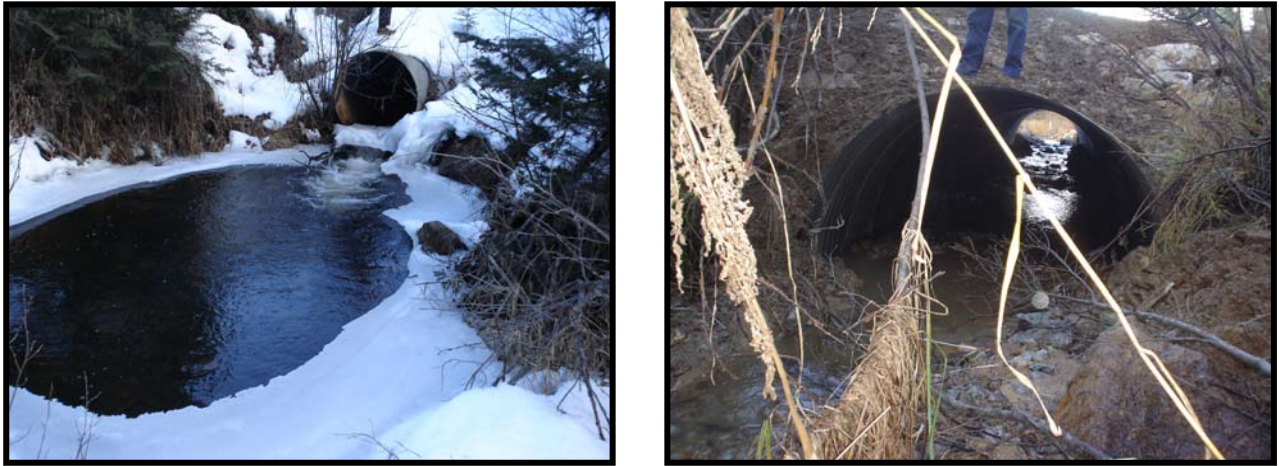
Figure 3. Outlet of the Weaver Creek culvert replacement before and after.
