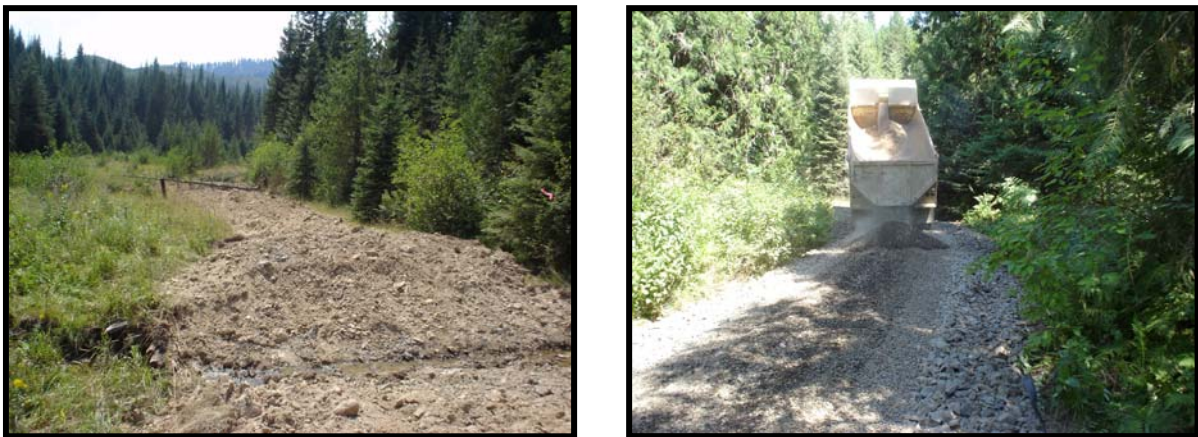
Figure 3. Typical road obliteration at Blonde Creek and road improvements at Lolo Creek..
