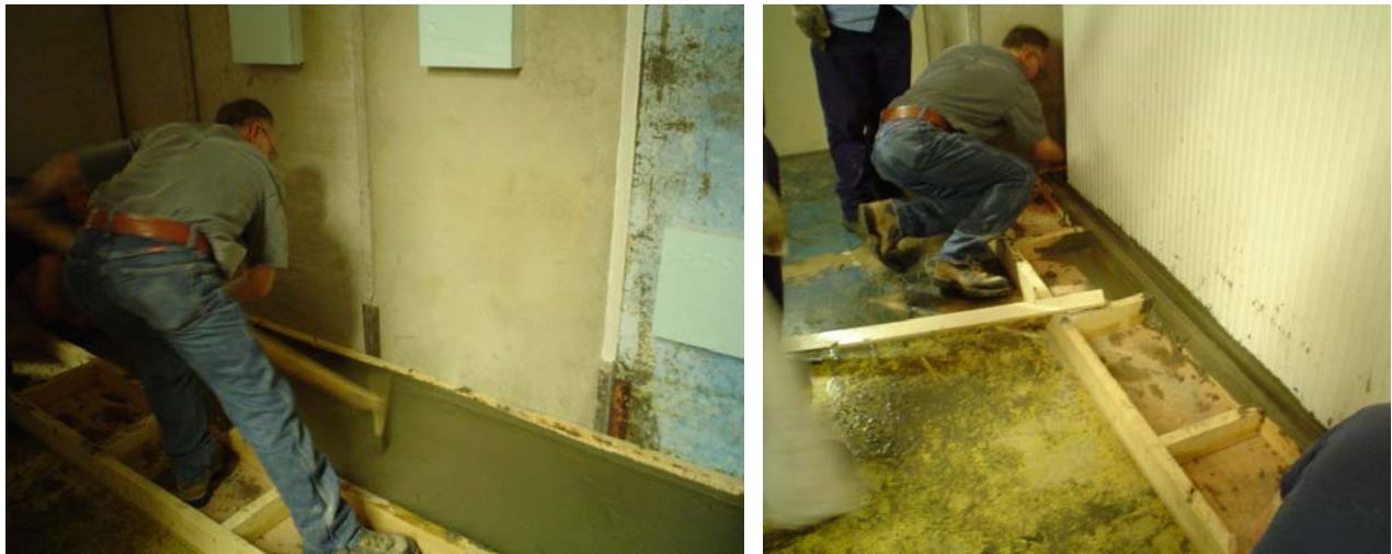
Figure 2: Grout the IPND prototype
