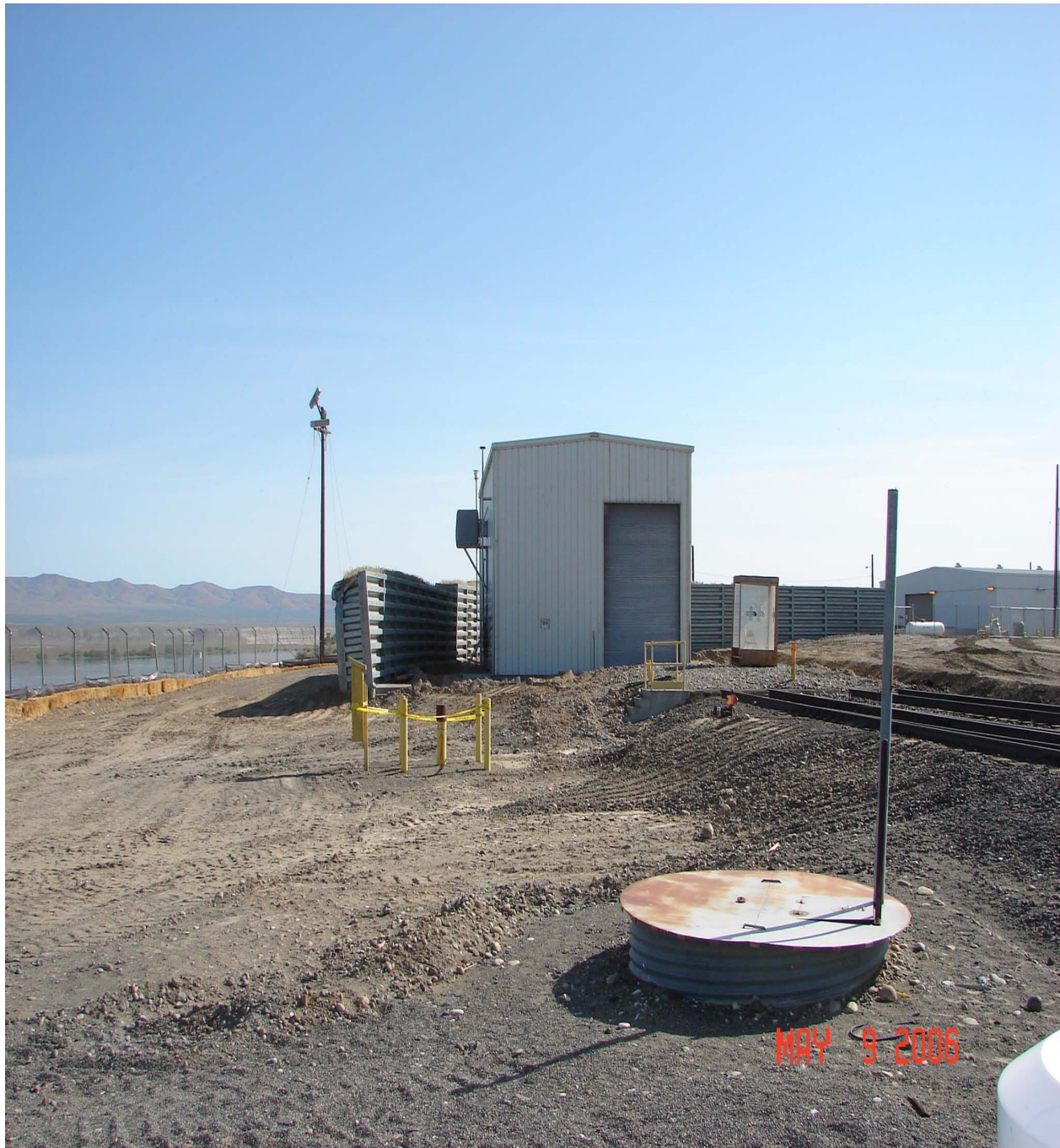
Figure 5. 1314-N liquid Waste Loadout Station.
