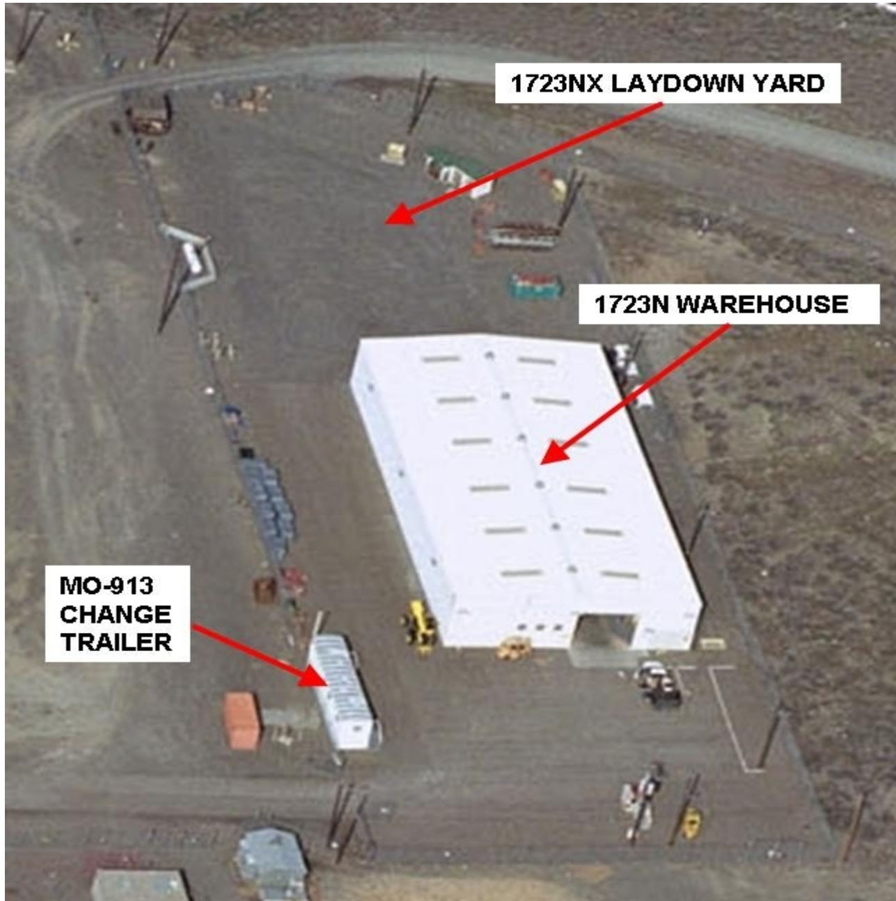
Figure 9. 1723-N Warehouse, 1723-NX Laydown Yard, and MO-913 Change Trailer.
