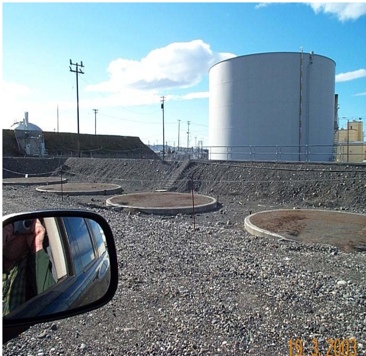
Figure 3. 1715 Fuel Oil Storage Tank Foundations 1-5.
