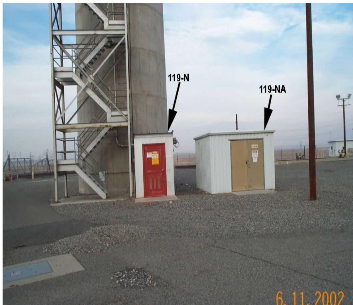
Figure 6. 119-N/NA Air Sampling and Monitoring Facilities.
