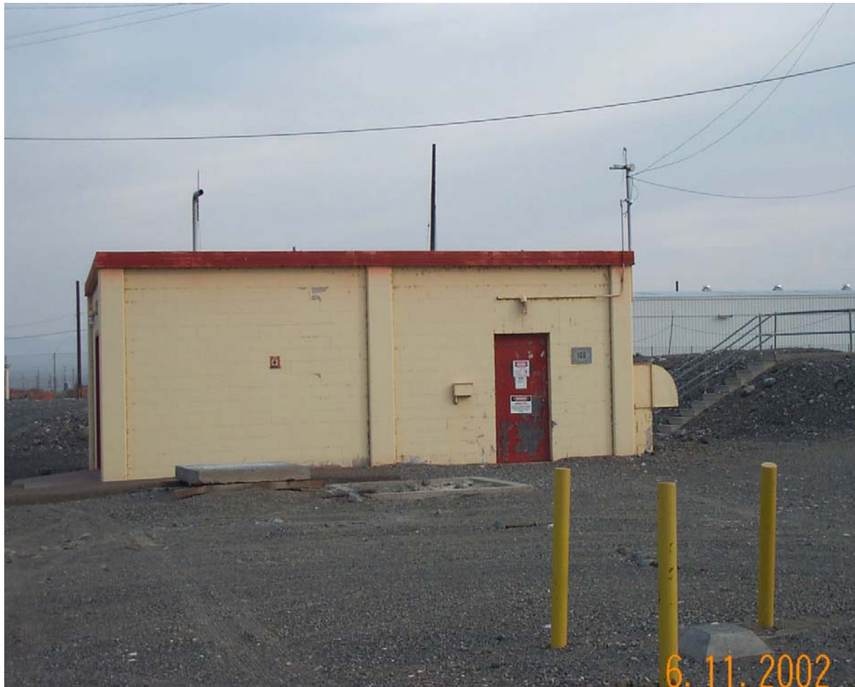
Figure 2. 166-N Fuel Oil Pump House/Unloading Station.
