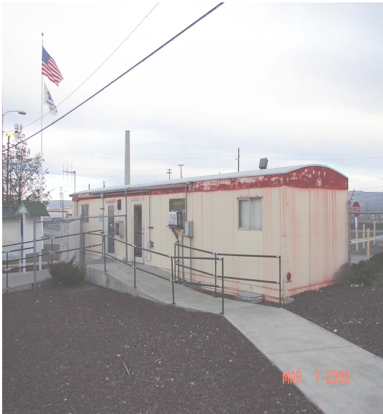
Figure 7. 1701-N Limited Access Area Badge House.
