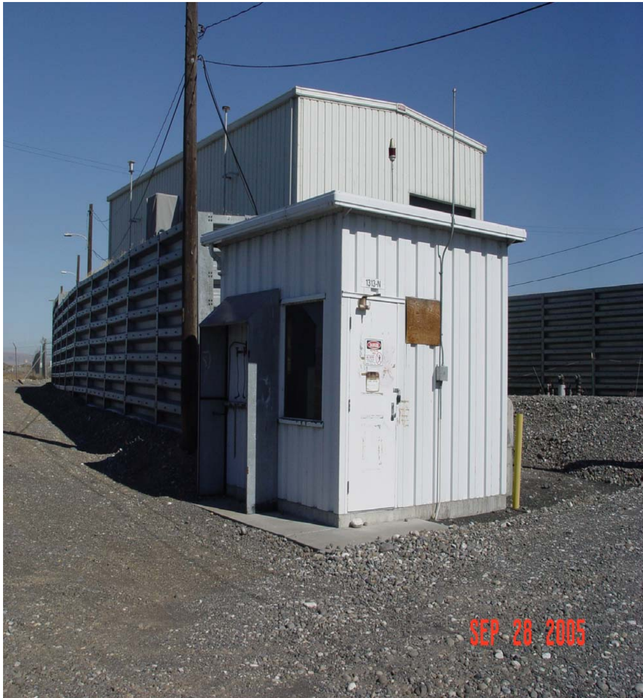
Figure 4. 1313-N Change Control Room.
