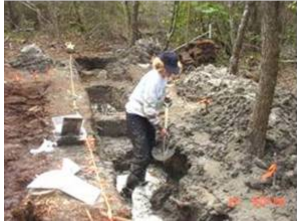
Figure 10. Slurry of soil and water made for difficult excavation.
