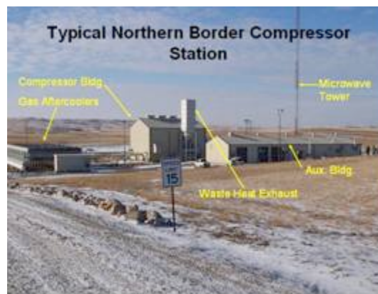
Figure 23. Compressor Station Overview Pictures
