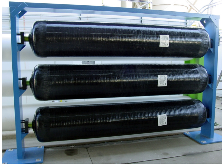
Figure 28: GTI Three Bank Cascade With Composite Pressure Vessels
