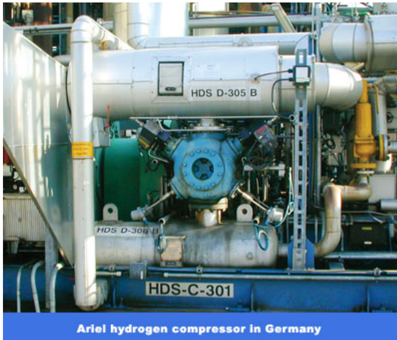
Figure 40: Larger Hydrogen Reciprocating Piston Compressor
