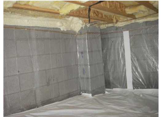
Complete Wall Liner
