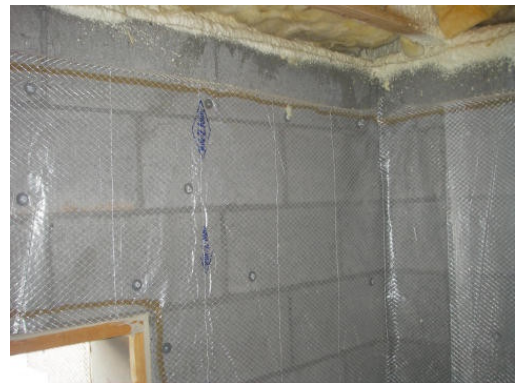
Liner Sealed to Block Wall
