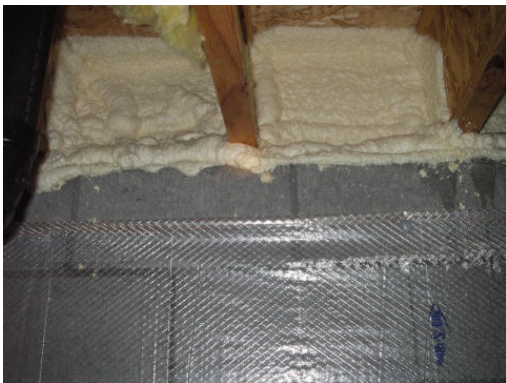
Air Sealing Band Joist
