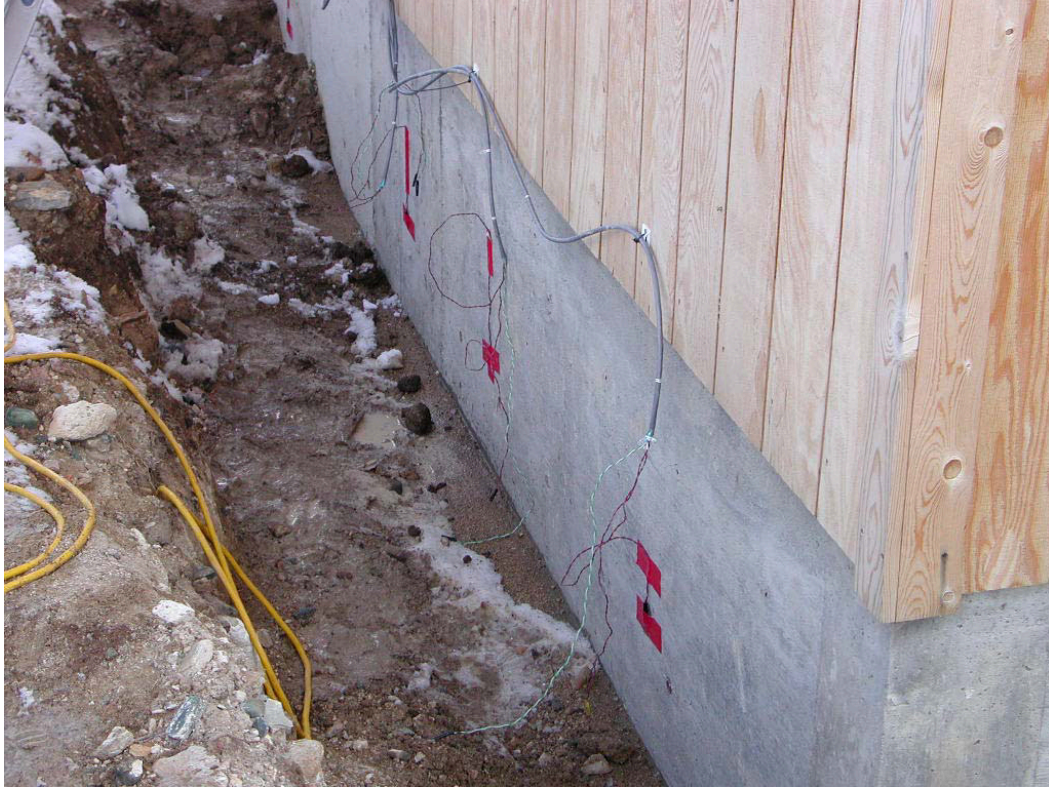
Figure 8. Temperature sensors installed on outside surface of foundation.
