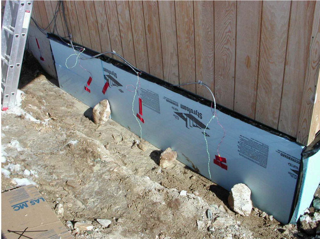
Figure 9. Temperature sensors installed on outside face of insulation.
