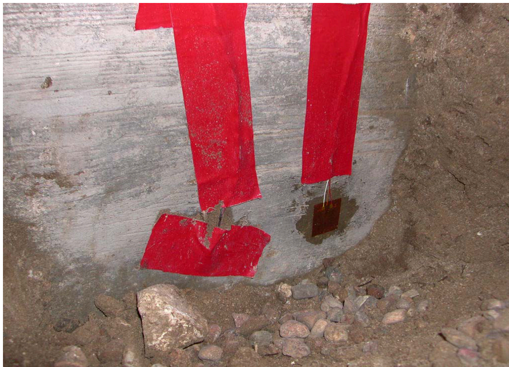
Figure 7. Temperature sensor and heat flux sensor as placed on foundation interior
