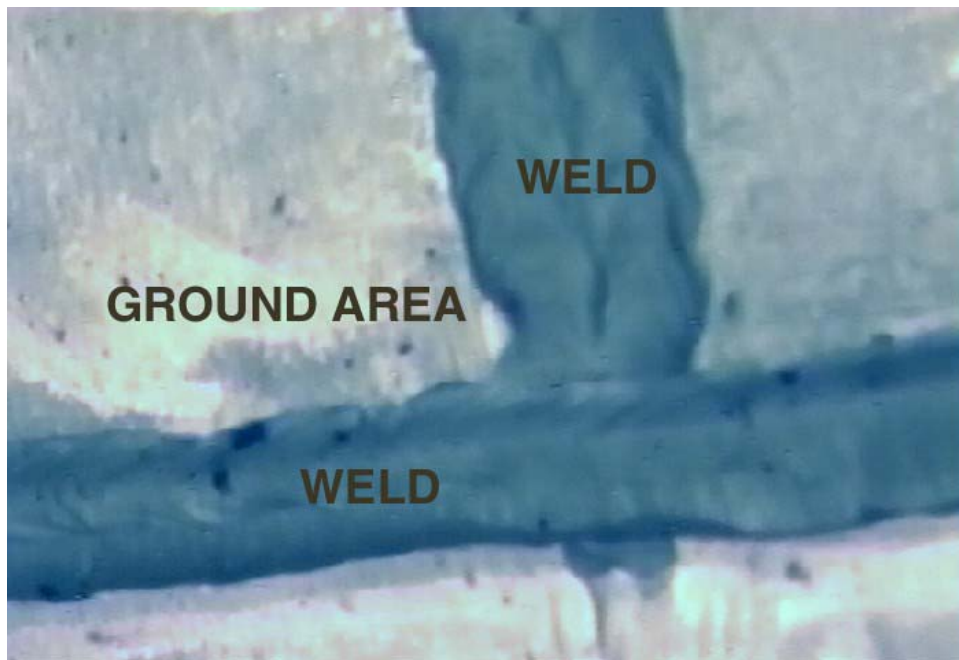
Figure D-4. Weld intersection in Tank WM-188 (PD03-0029-05). 5
