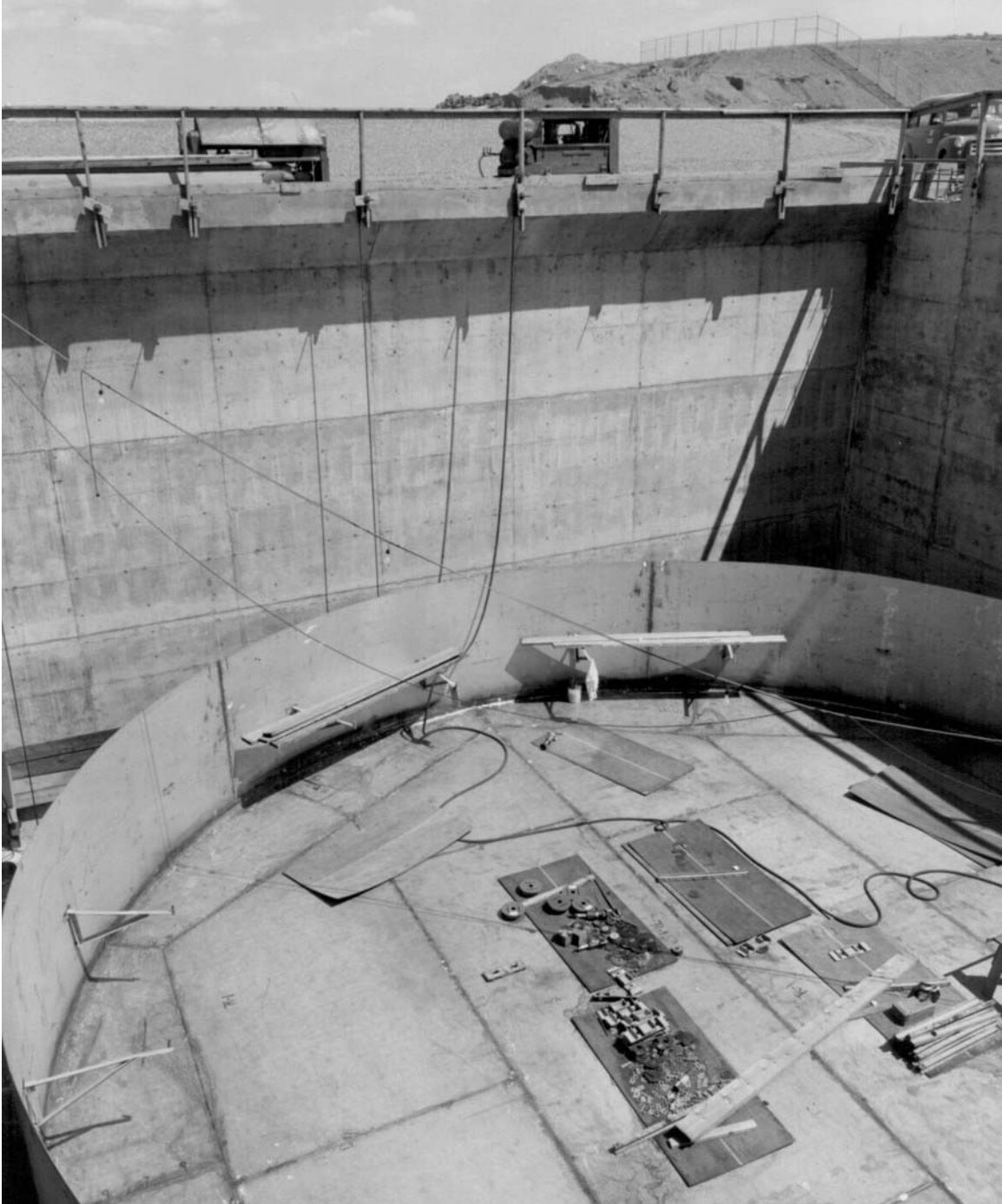
Figure D-1. Construction of Tank WM-188 (58-3473).
