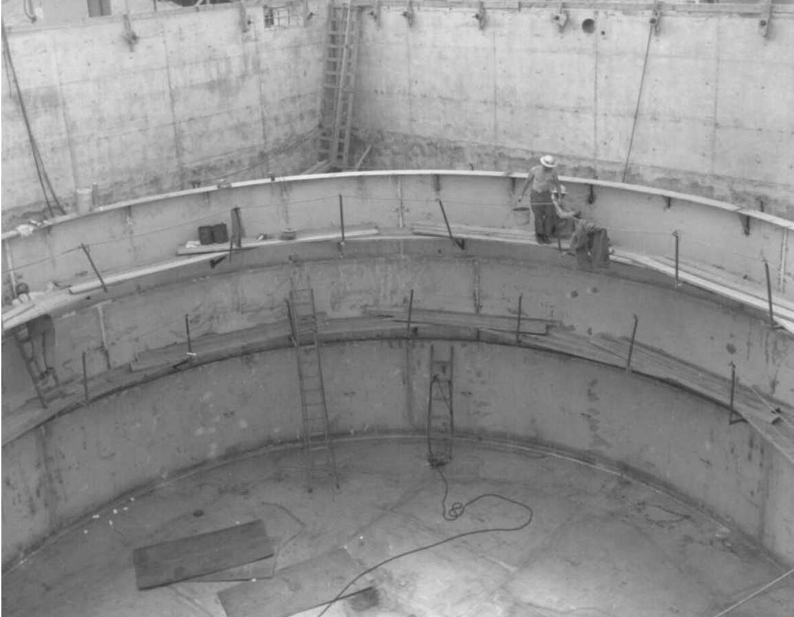
Figure D-2. Later stages of construction of Tank WM-188 (58-4236).
