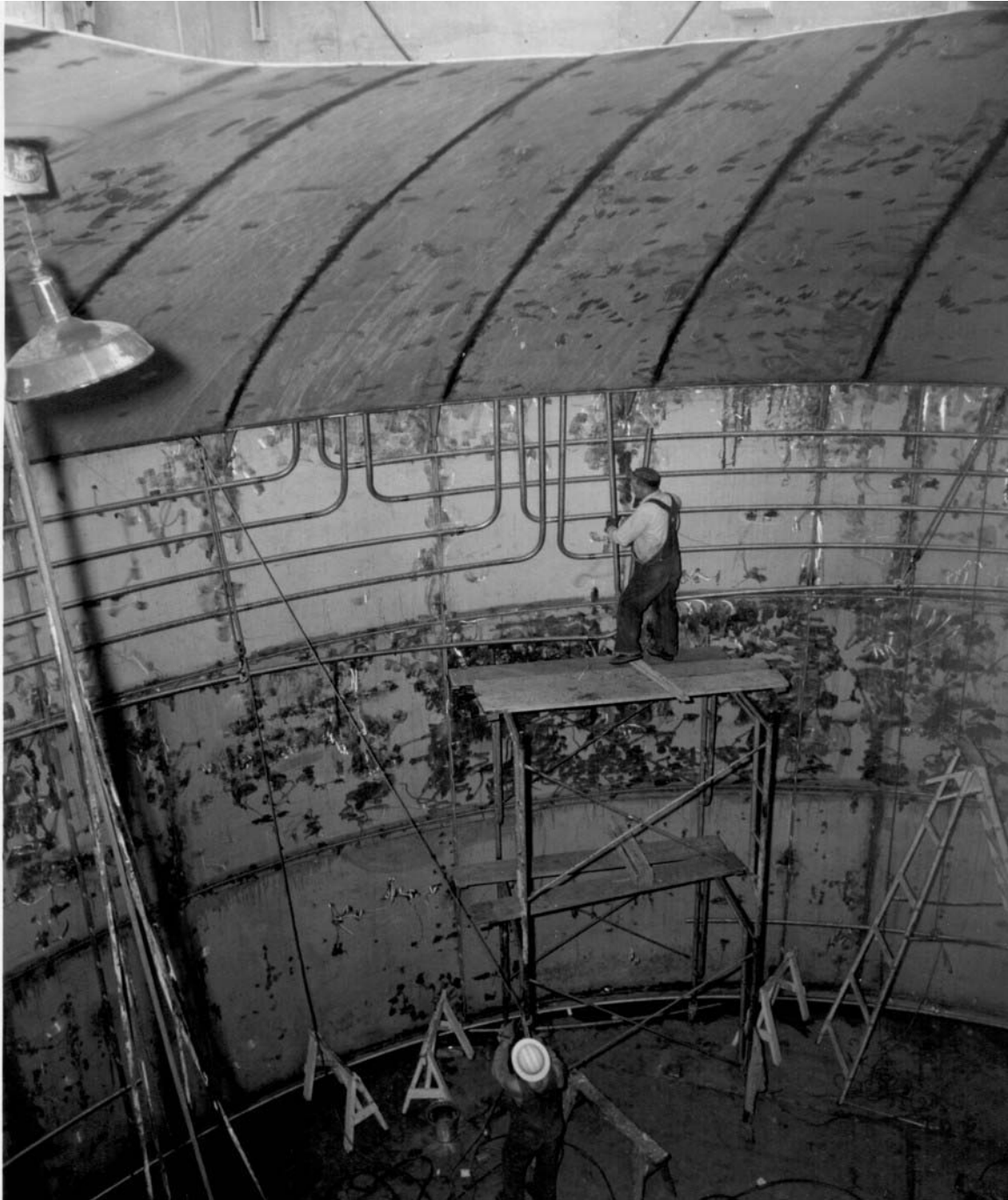
Figure D-3. Installation of cooling coils for Tank WM-187 (58-4237).
