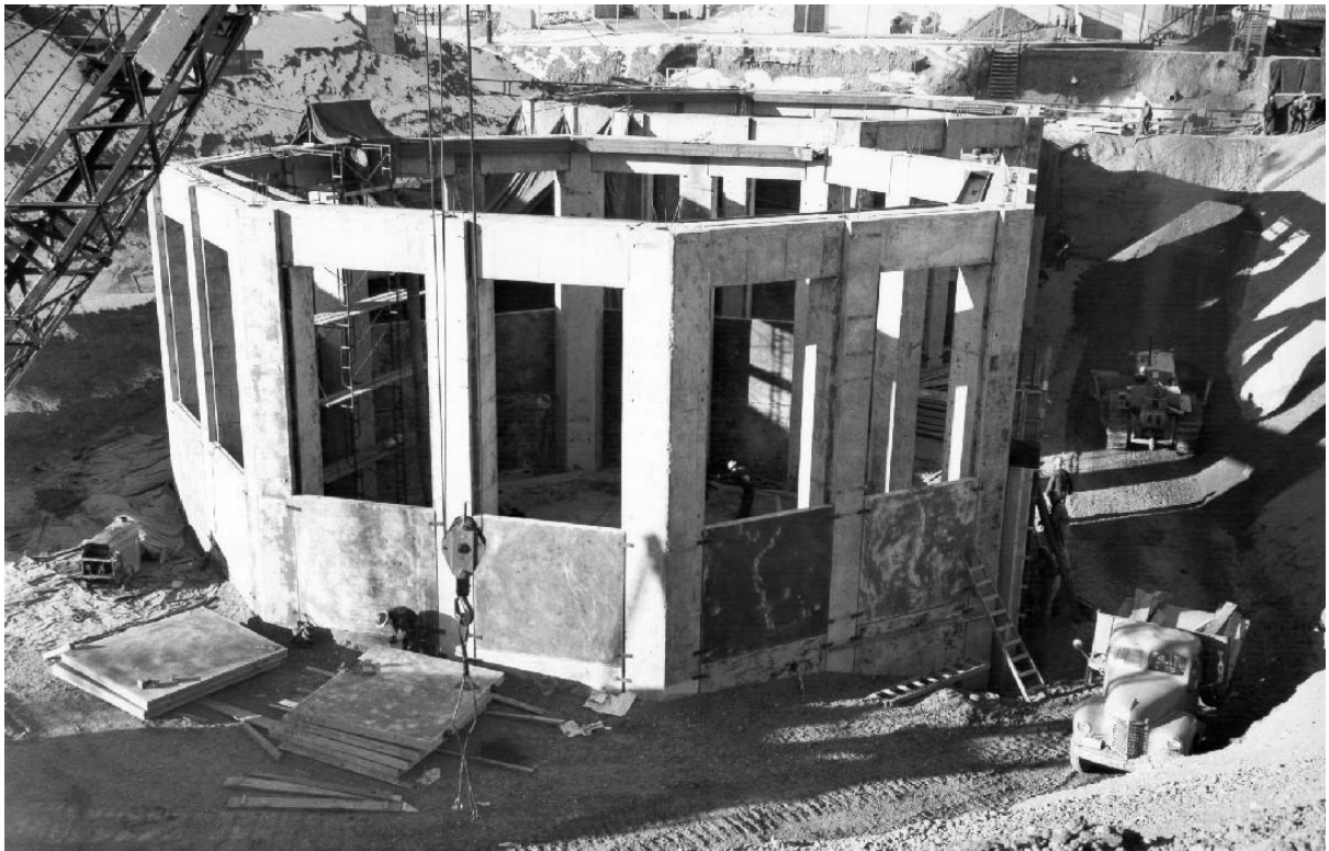
Figure 5. Octagonal, pillar-and-panel vault for Tanks WM-182 and -183, and the type used for Tanks WM-183, WM-185, and WM-186 (13450).
