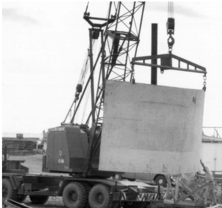
Figure D-6. Hoisting of plate section showing lifting device (63-6763). 5
