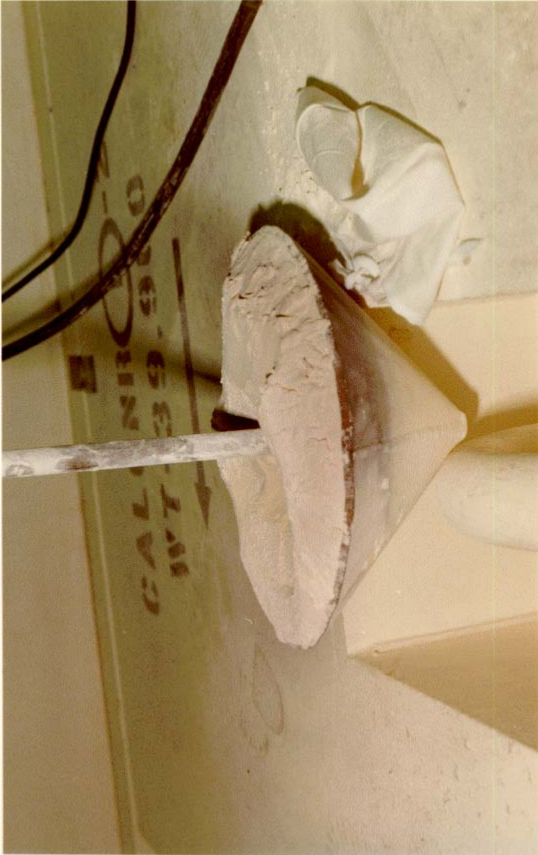
Figure A-5. Calciner baffle inspection port plug filled with calcine before decontamination (81-5584).
