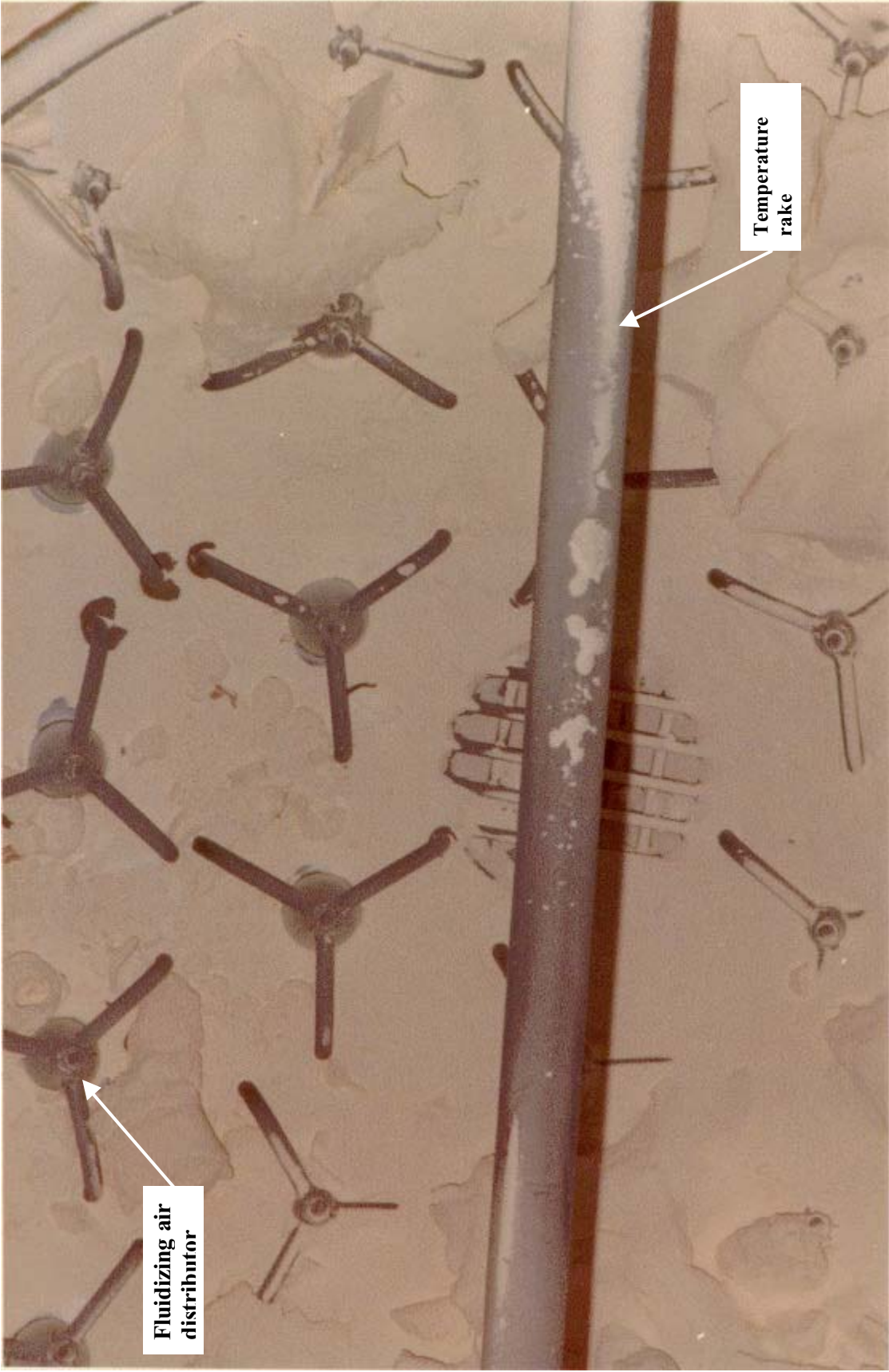
Figure A-7. Close-up view of calcine on top of fluidizing air distributor plate prior to decontamination. Several fluidizing air distributor caps with their three support legs are visible and others are covered with calcine. Varying amounts of calcine cover the distributor caps (81-5593).
