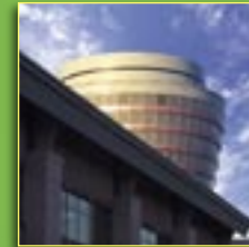
More than 60 percent of the heating and cooling at Lansing Community College's West Campus is provided by a geothermal system, which extracts heat from the earth. The system saves the college about $100,000 in energy costs per year.
