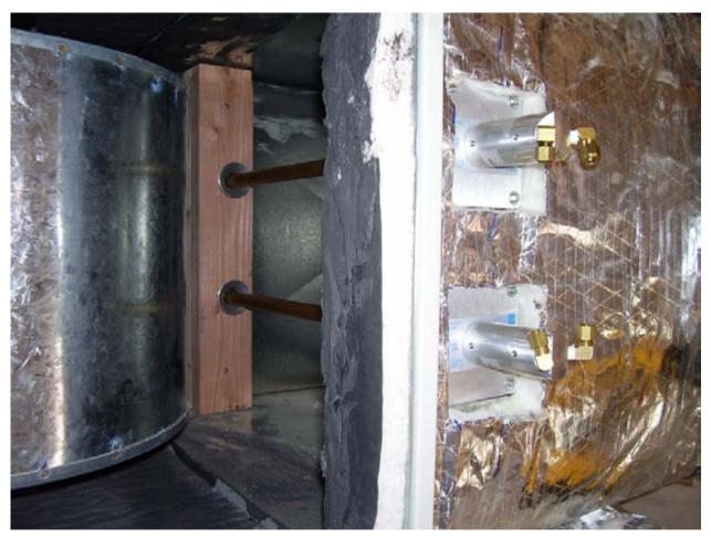
Figure 23. Pitot tube traverse airflow sensors installed at the return duct for the DiGiorgio home
