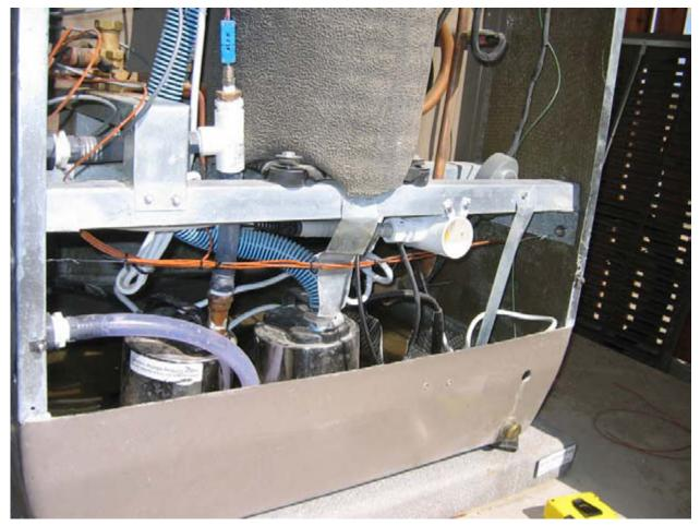
Figure 26. Thermocouple (brown wire) and Vaisala temperature and RH sensors (white PVC shield + gray sensor) installed at Freus air intake, grill removed
