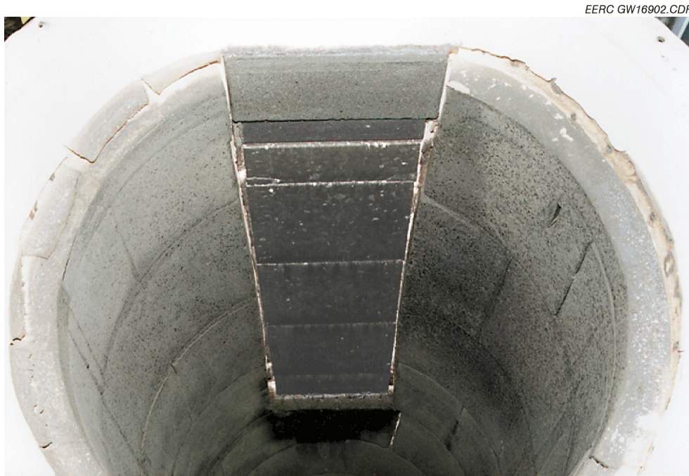
Exhibit 11-63 Photograph of the Monofrax M Tiles Inside the Furnace Following SFS Test SFS-RH10-0699
