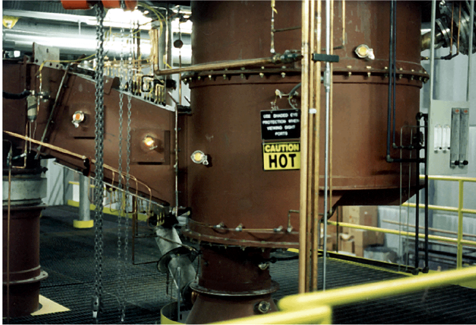
Exhibit 11A-6 Photograph of the Two Lower Furnace Sections
