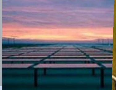
Shell Solar at Semitropic Water S 980 kW, single-axis tracking, Was
