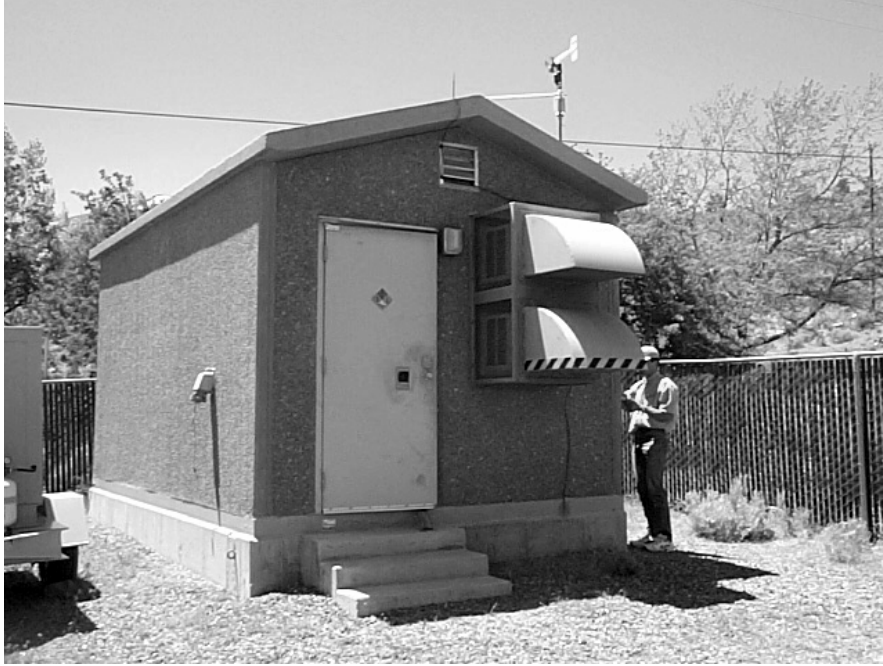
Figure 1: Typical Regen Building.
