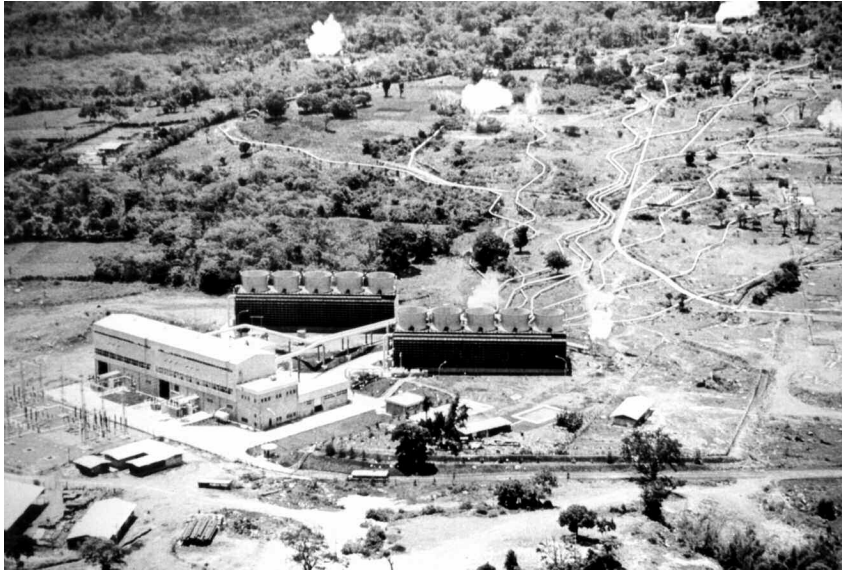
Figure 8.2 Ahuachapan geothermal facility after commissioning around 1977 (DiPippo, 1978).
