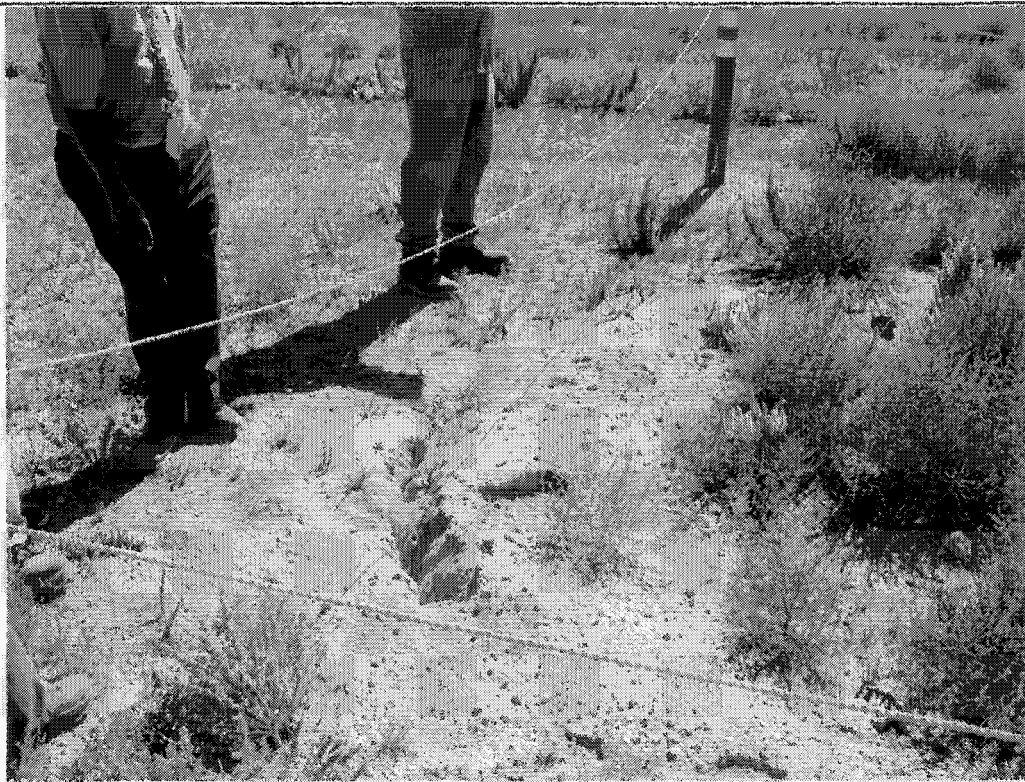
11. Subsidence area along southeast side of cover.
