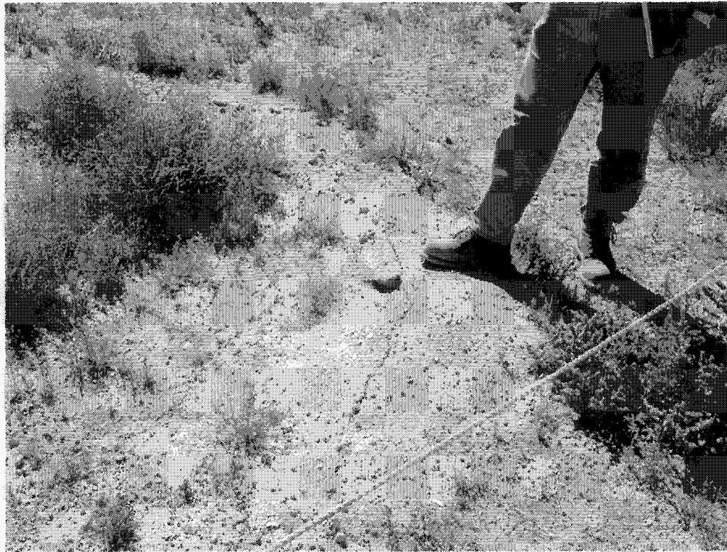
12. Subsidence area along southeast side of cover.
