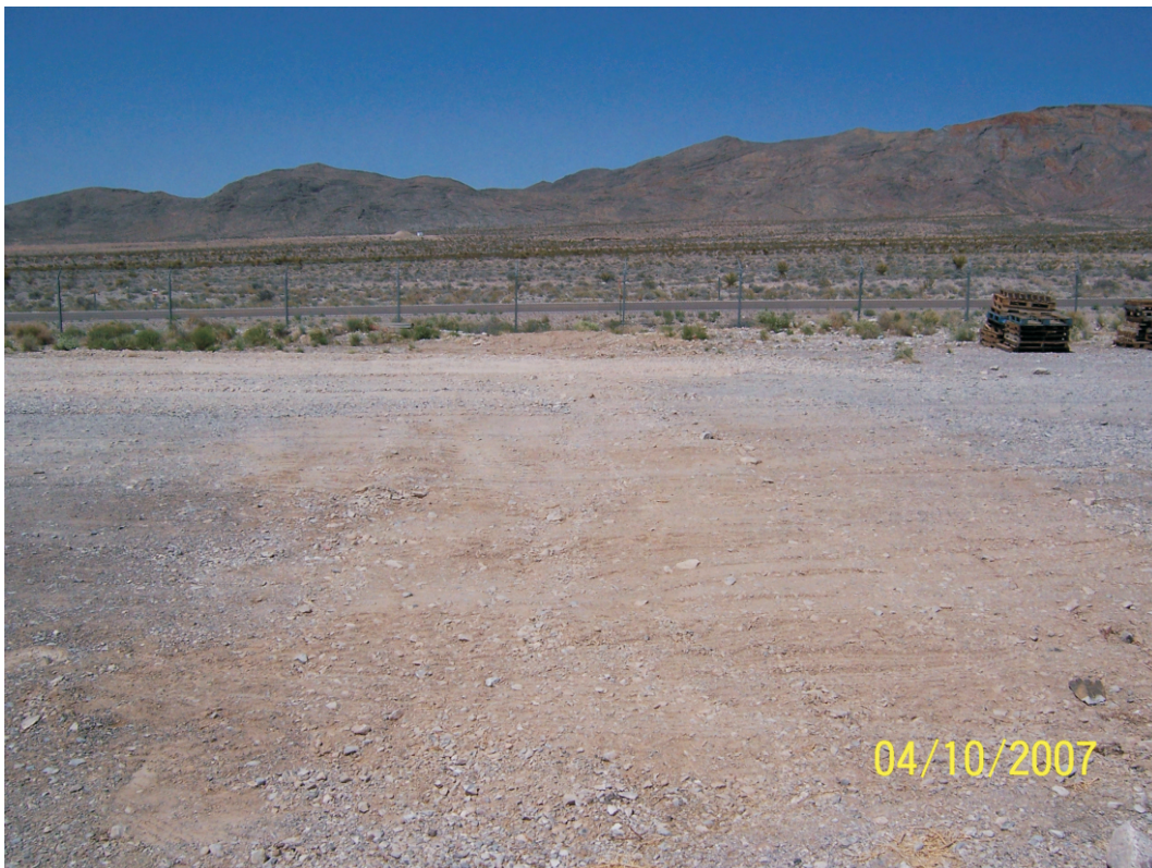
Photograph 2: CAS 23-25-02, Pipe location after pipe removal and backfill (04/10/2007)
