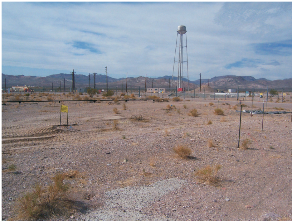
Photograph 6: CAS 25-60-01, South area after excavation and backfill (08/14/2007)
