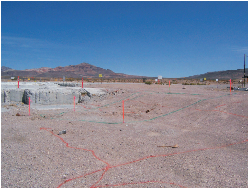
Photograph 3: CAS 25-60-01, North area prior to excavation (04/19/2007)
