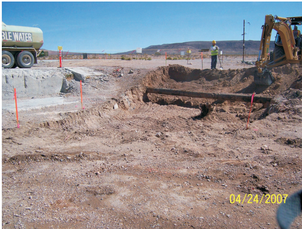
Photograph 4: CAS 25-60-01, North area during excavation (04/24/2007)
