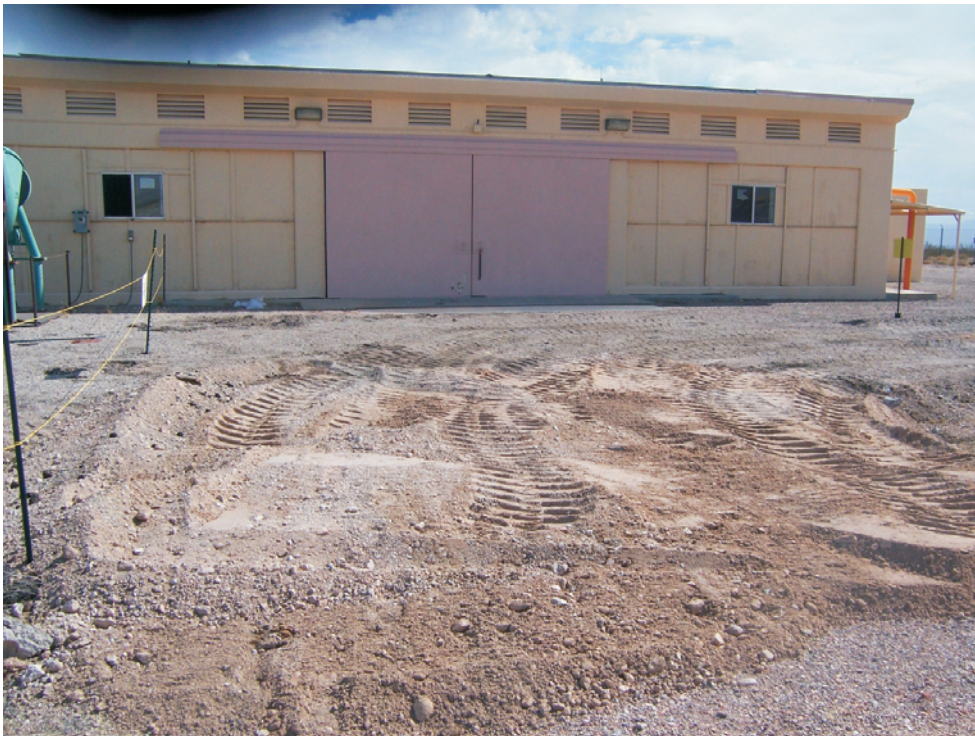
Photograph 8: CAS 26-62-01, Soil location after excavation and backfill (08/14/2007)
