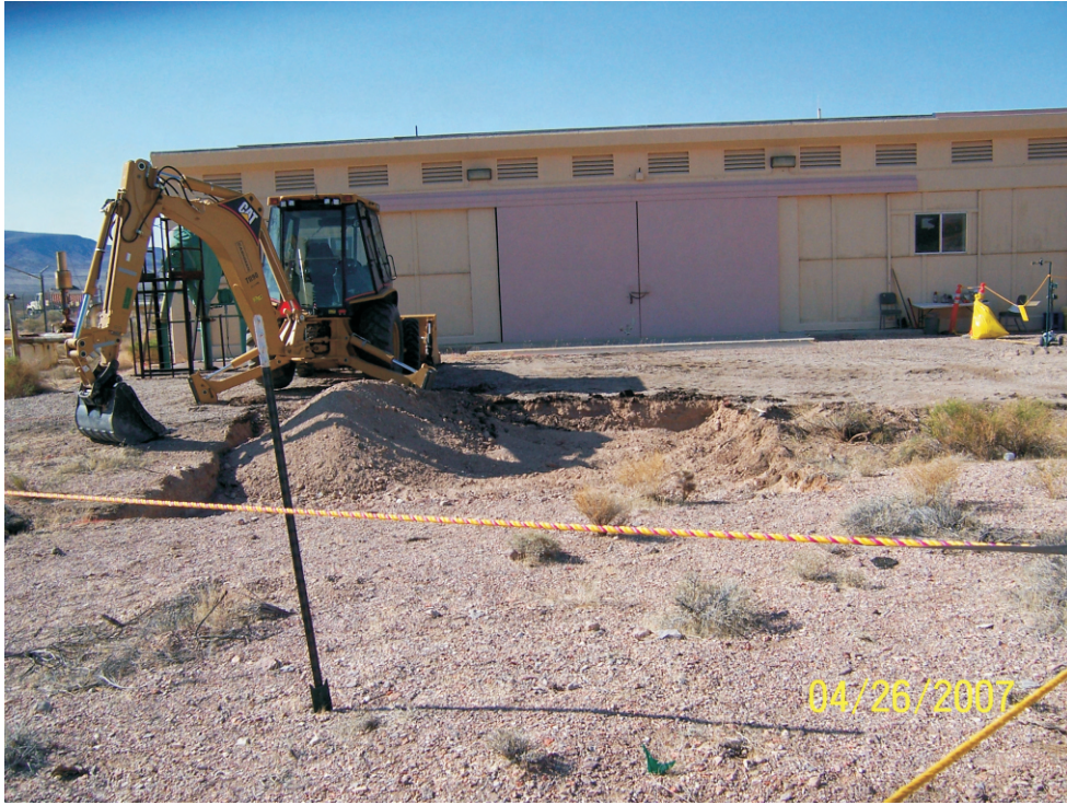
Photograph 7: CAS 25-62-01, Soil location during excavation (04/26/2007)
