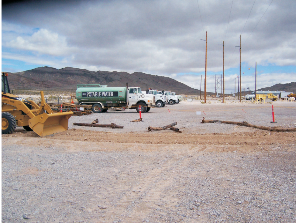
Photograph 1: CAS 23-25-02, Pipe location during pipe removal (03/21/2007)
