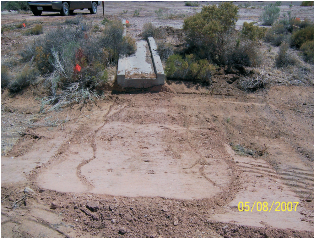
Photograph 9: CAS 26-60-01, Soil location after excavation and backfill (05/08/2007)
