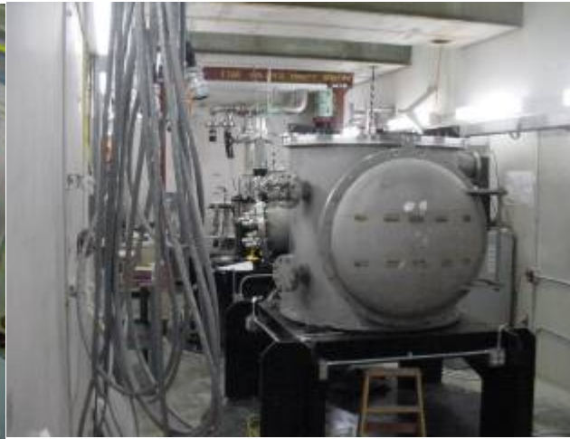
Flywheel test chamber
