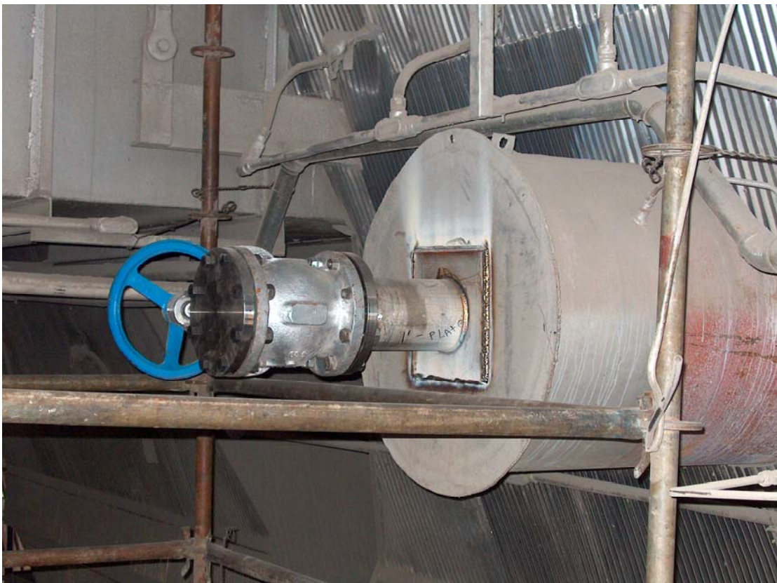
Figure 43. Outlet port installed at air preheater exit at Plant Gadsden.
