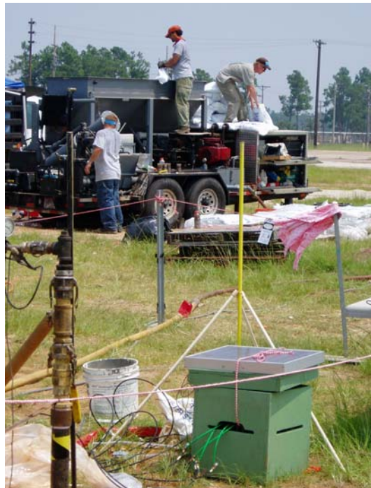
Figure 6 – Well Head and Fracturing Rig during Test
