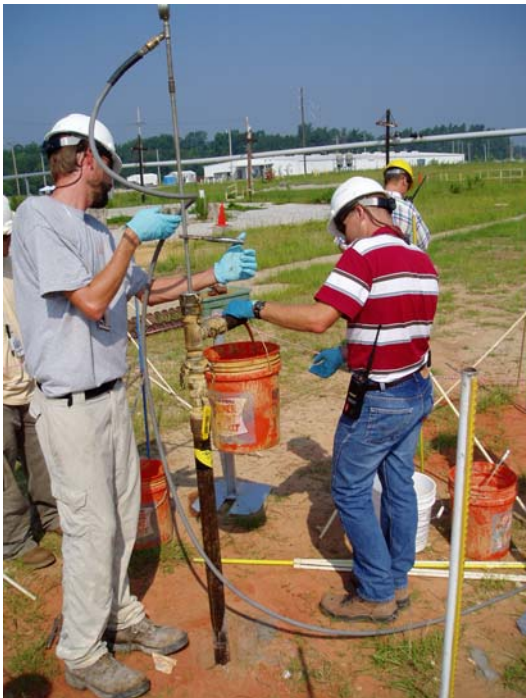
Figure 5 – Notching Well Prior to Hydraulic Fracturing
