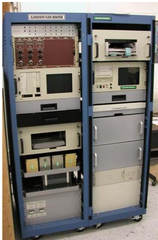
Fig. 9. The BDMS main cabinet housing the FMFM (left) and EM (right) cabinet sections.
